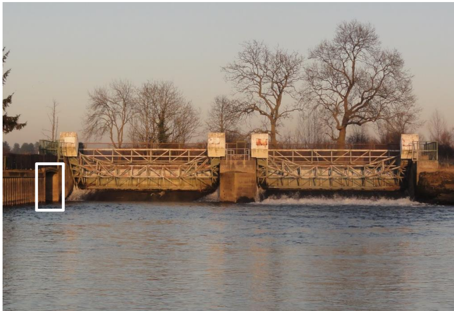
Figure 2.2. Elvington Sluices. The white outline indicates the location of the pool and weir fishway entrance. Photograph taken on 14/01/2012
