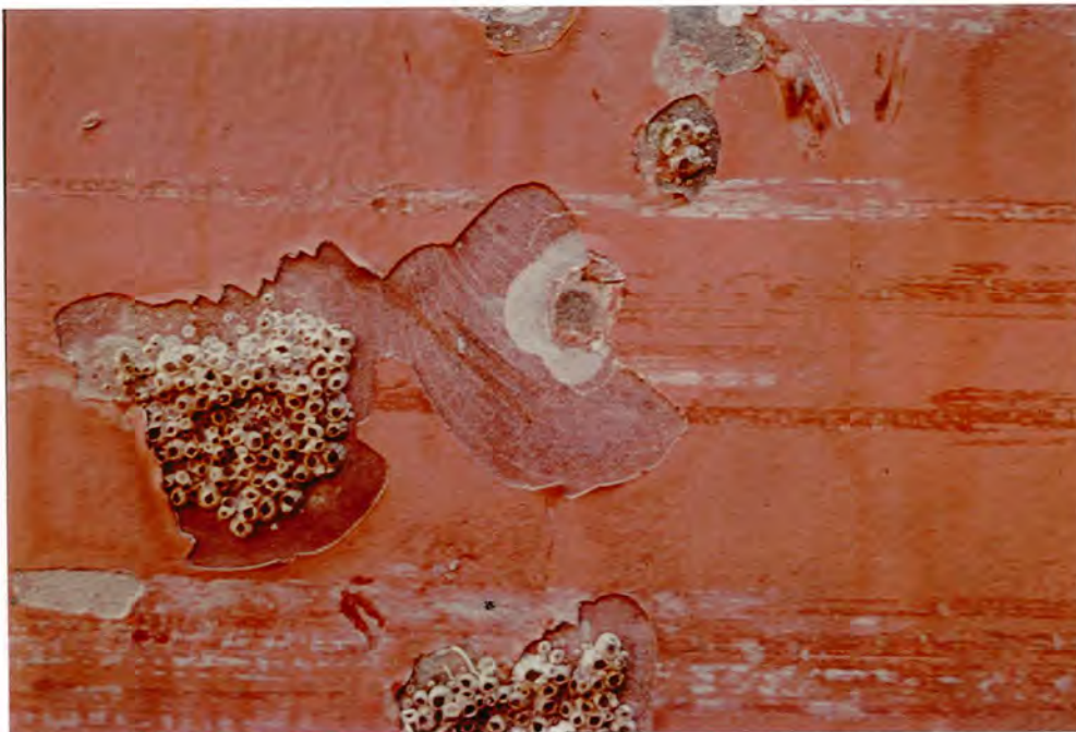
Figure 1.7 Typical barnacle fouling in regions of anti-fouling coating failure
