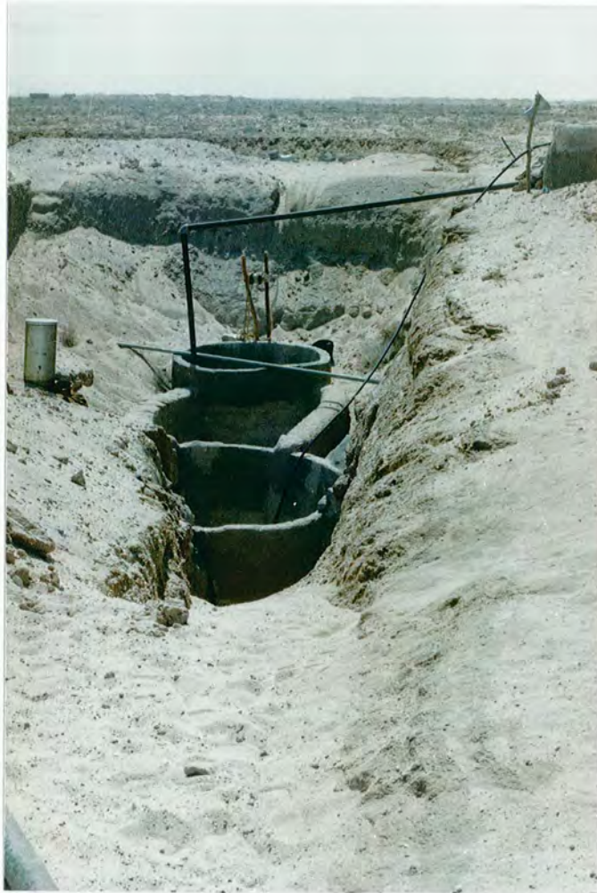
FIGURE 3.3 : Reconstruction of an old well
