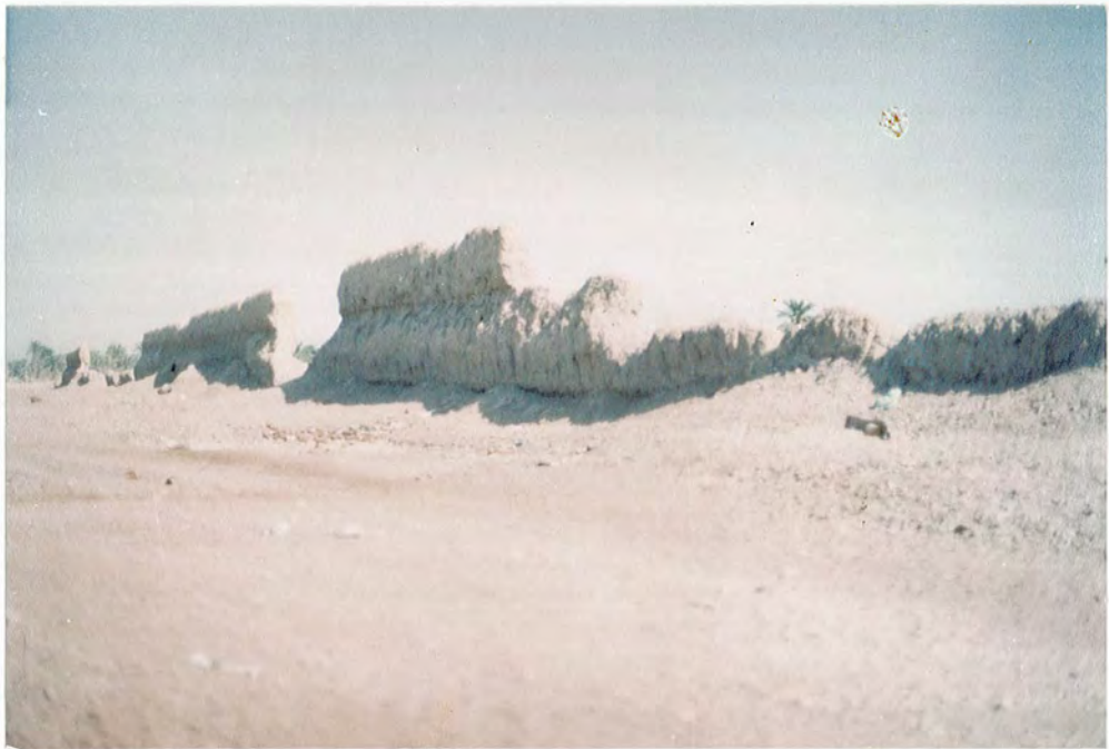
FIGURE 6.18 : The remnants of the earth embankment
