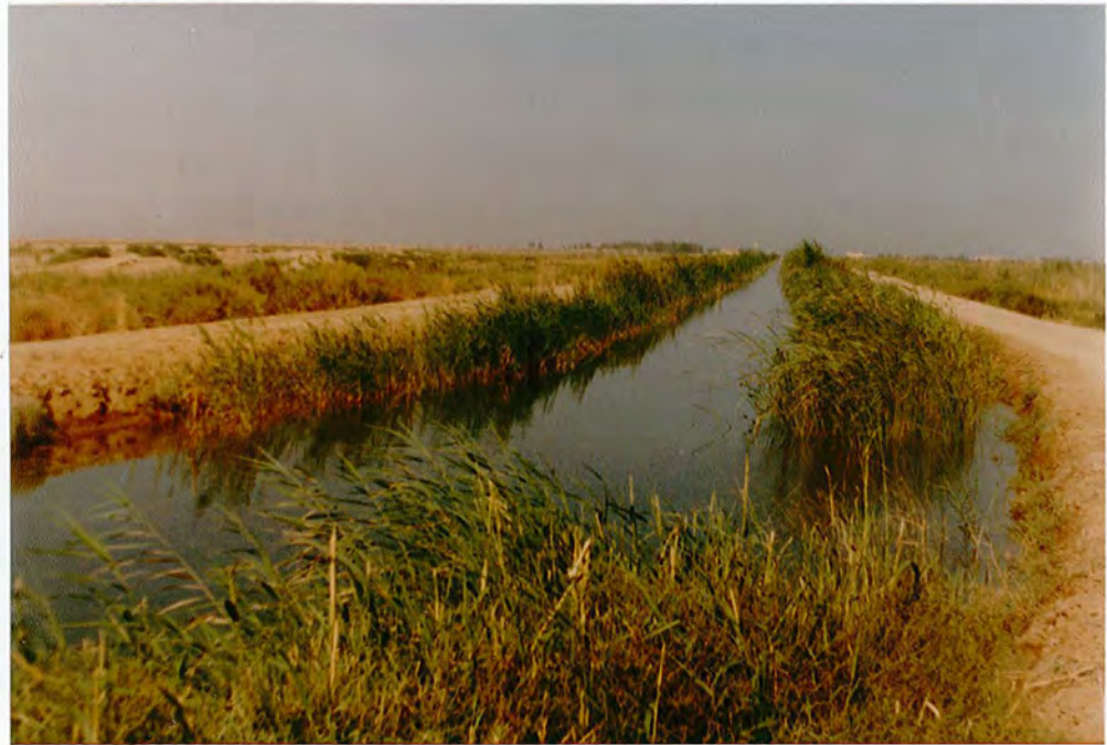
FIGURE 4.15 : The main canal and the weed growth depending on irrigation and seepage water
