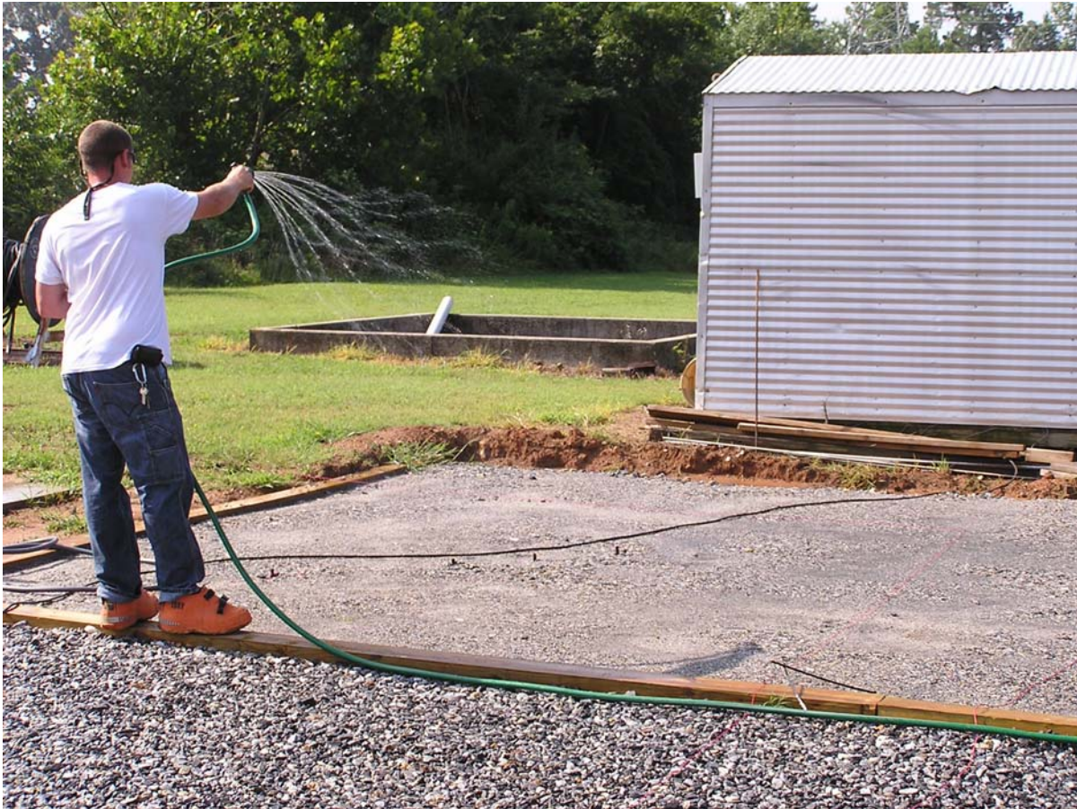
Figure 2-3 – Wetting of Test Area Prior To Testing
