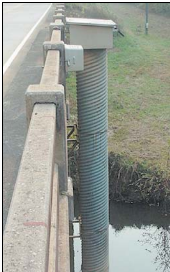
Figure 2. Typical flood-monitoring gage composed of a water stilling well and a gage house that shelters stage-recording equipment atop the stilling well.
