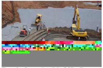
Figure 3. Construction of the RCC spillway steps using conventional earth moving equipment.
