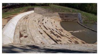
Figure 4. Completed Y-14 arced RCC spillway and ogee weir.
