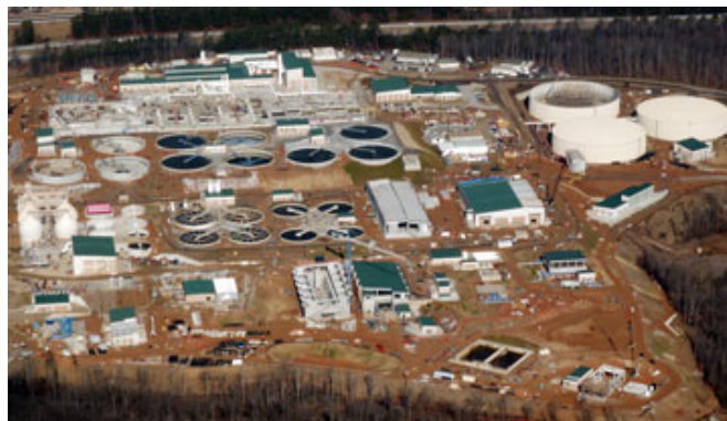
Figure 1. F. Wayne Hill Water Resources Center in Gwinnett County
