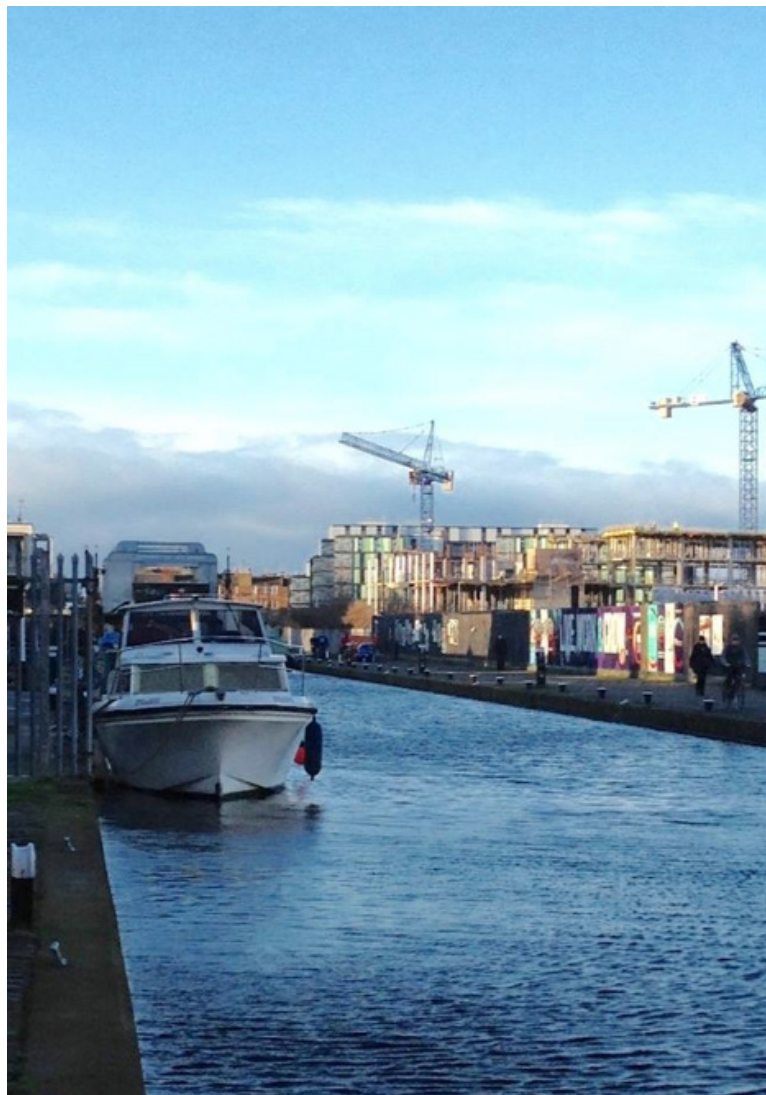
FIG 1: Construction on the canalside All photos © Authors
