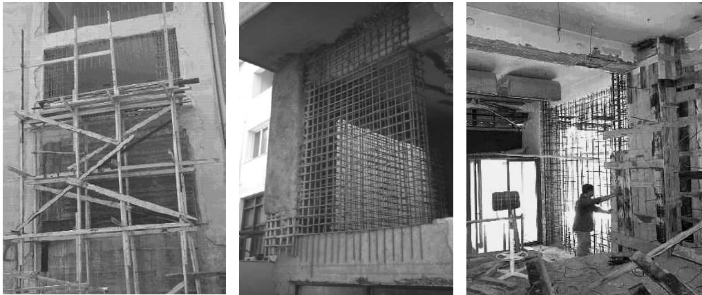
Fig. 5 Cast-in-place infill walls
