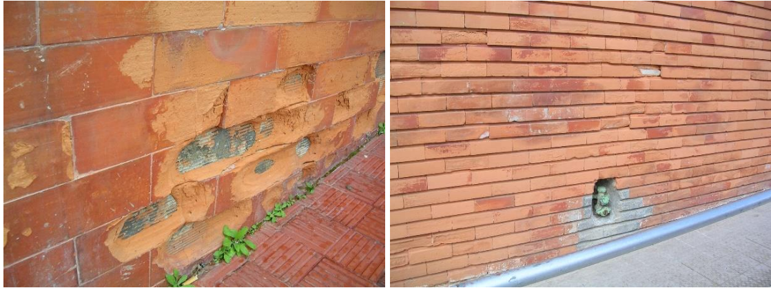
Figure 9. Illustrative example of the pathological situation of a case study located less than 5 km from the sea.
