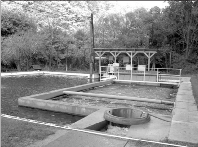
Figure 4. The view of the biological filter at the “Hoitsy and Rieger” intensive trout farm
