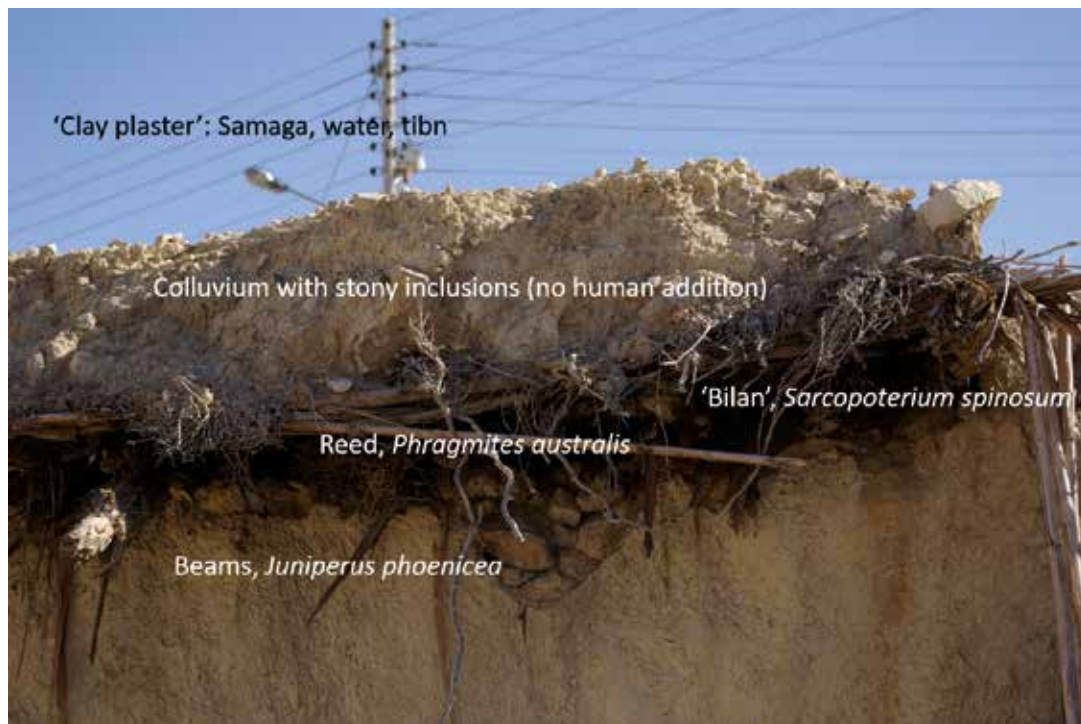
Fig. 5. Roofing materials from one of the houses at Al Ma'tan. Showing the different components used in roof construction: Juniperus phoenicea beams, Phragmites australis (reeds), 'Bilan' ( Sarcopoterium spinosum ), colluvium and clay plaster made from samaga (clay), tibn (temper) and water.
