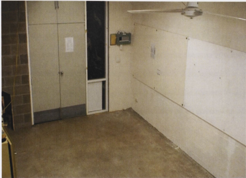
Figure 98: Overview of installation space as seen from rear corner.
