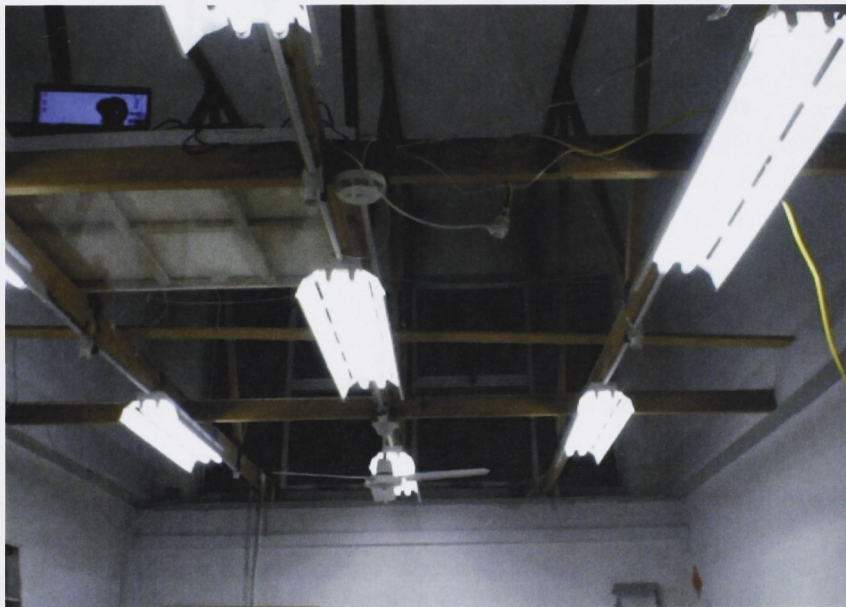
Figure 99: Overview of the frame structure present within the ceiling space.
