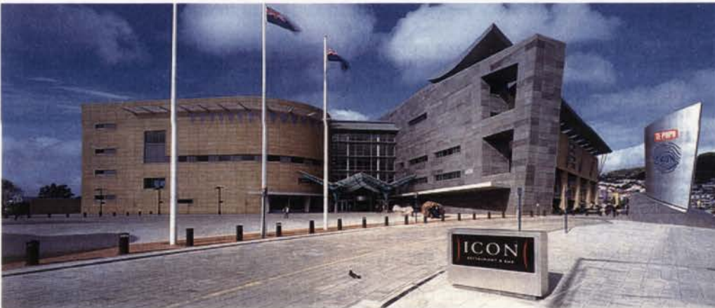
Figure 48 Front elevation of Te Papa. (Postcard Museum of New Zealand Te Papa Tongarewa)
