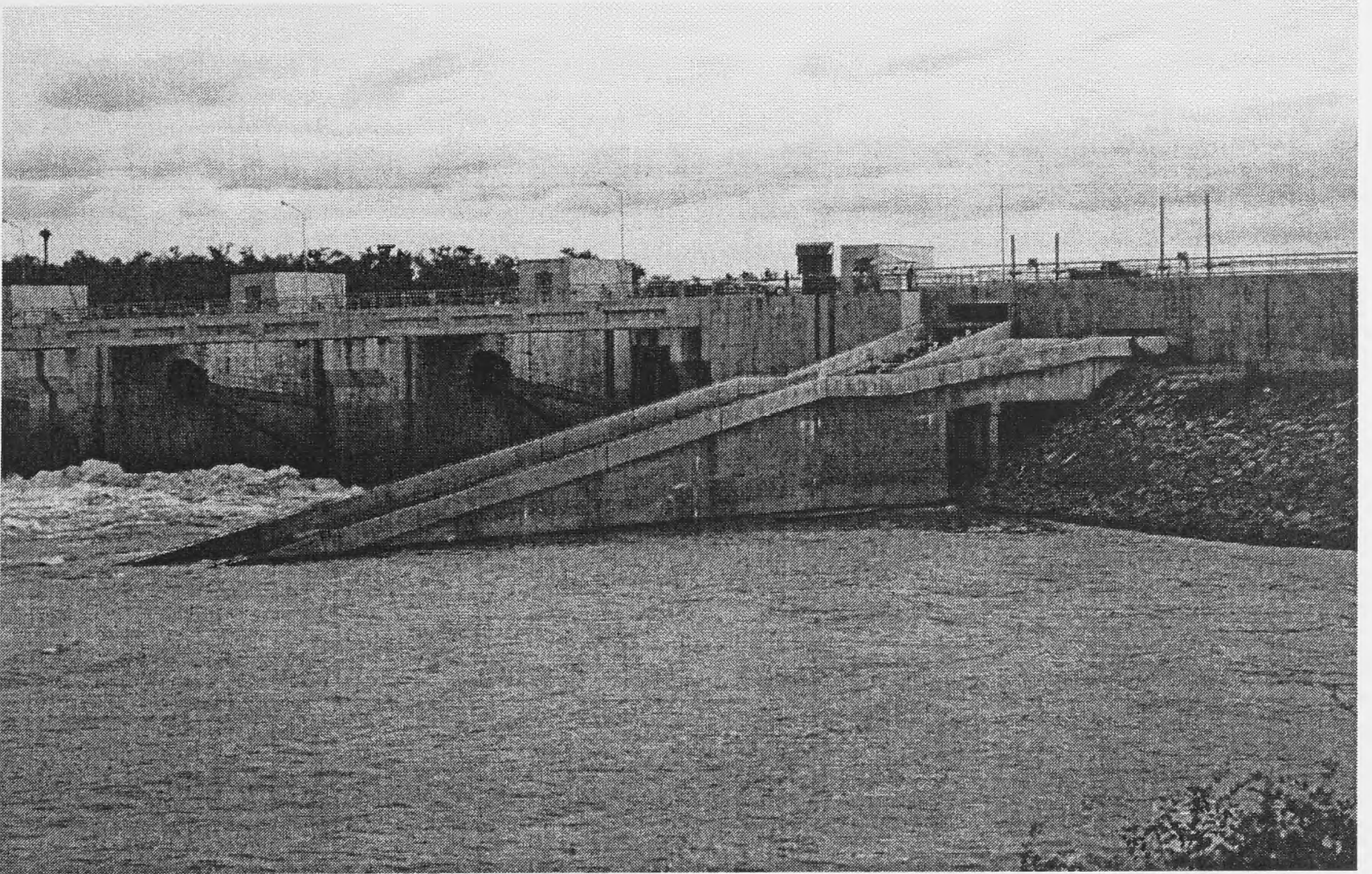
Photograph 3. The Pak Mun Dam wall and fish ladder that was added on to it in 1995. Local people declare “Thai fish can’t jump!”
