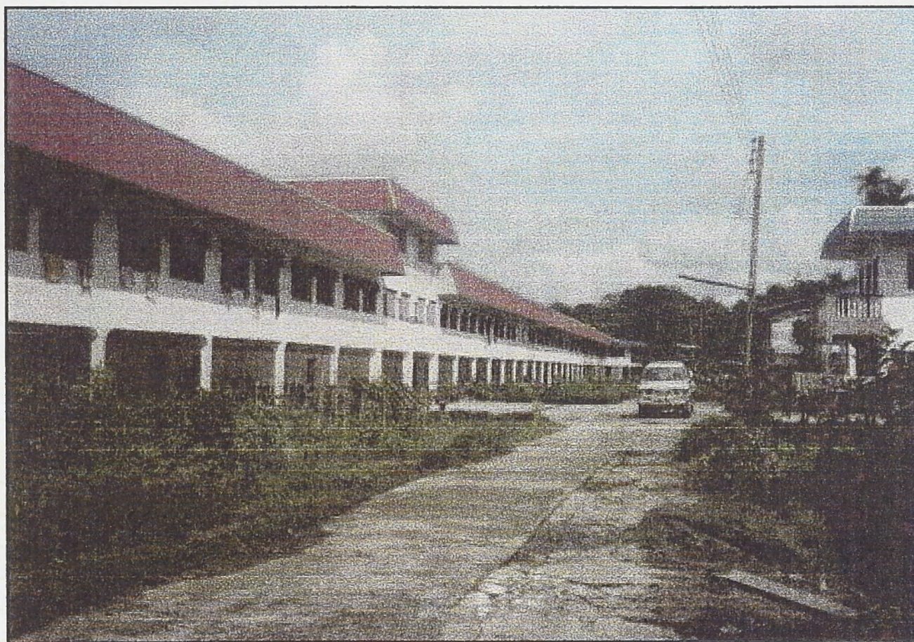
Figure 5: The new longhouse at Long Laput
