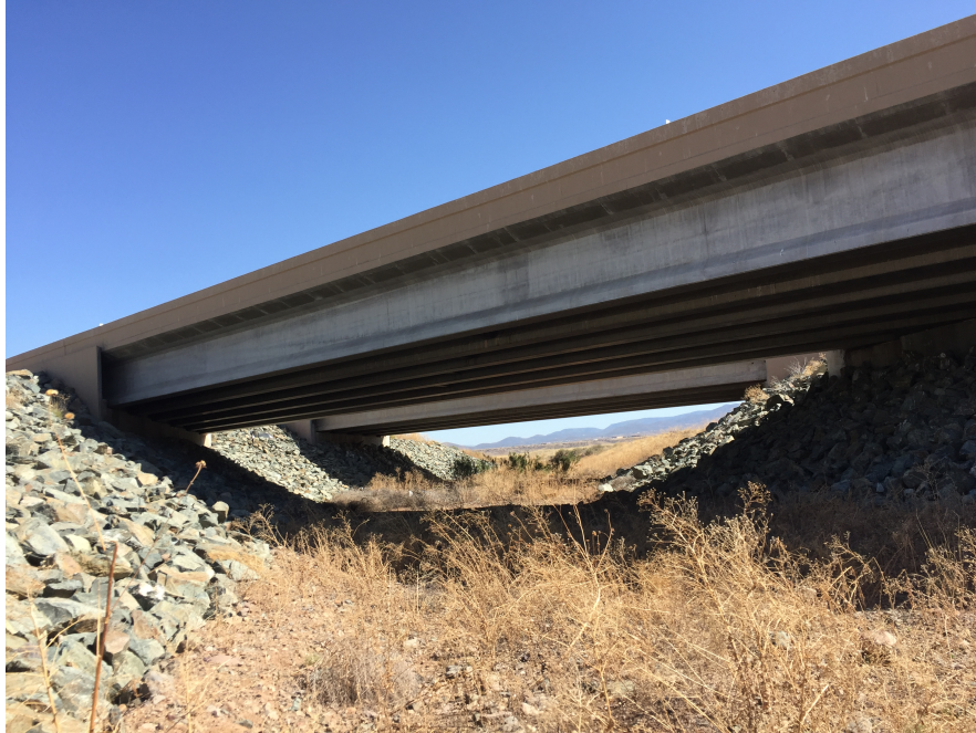
Figure 4-1: Coyote Wash Bridge
