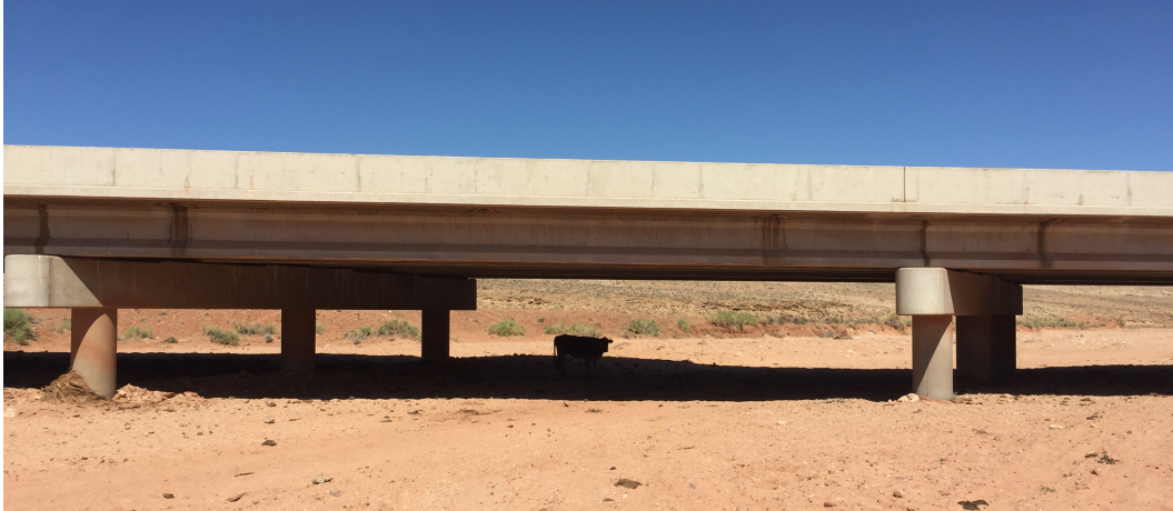
Figure 4-2: Tanner Wash Bridge
