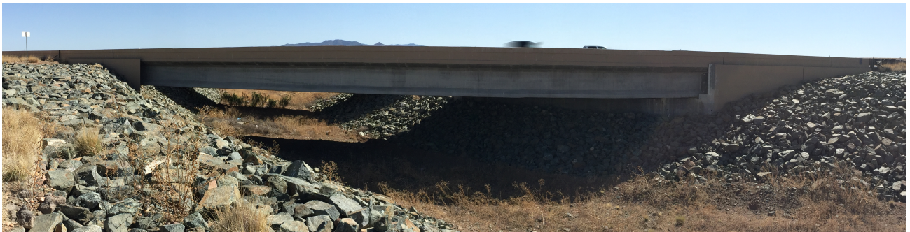
Figure 3-6: Coyote Wash Bridge
