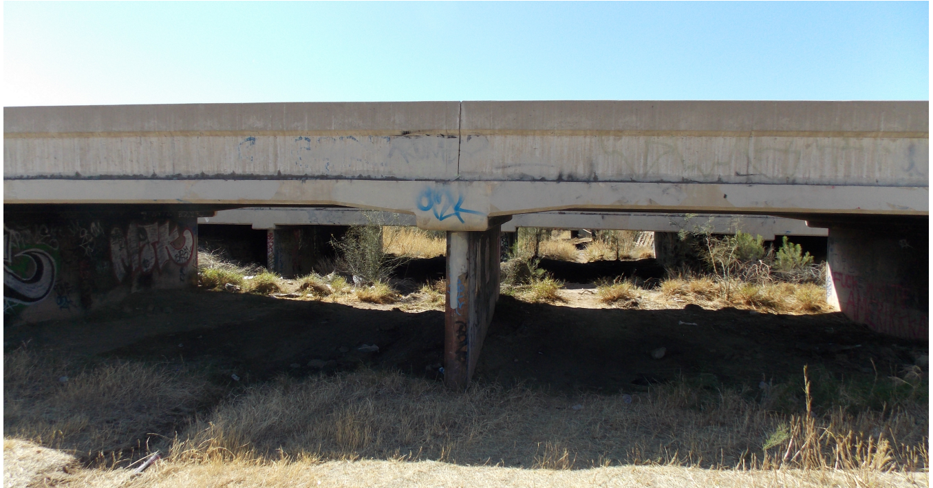
Figure 4-3: Earp Wash Bridge
