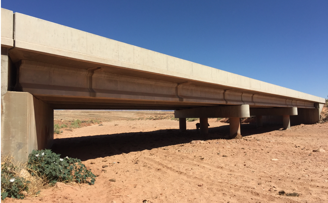
Figure 3-8: Tanner Wash Bridge
