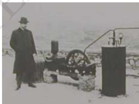
Fig. 8. Piero Ginori Conti and the 10 kW experimental power plant, Larderello, Italy, 1904 [42]
