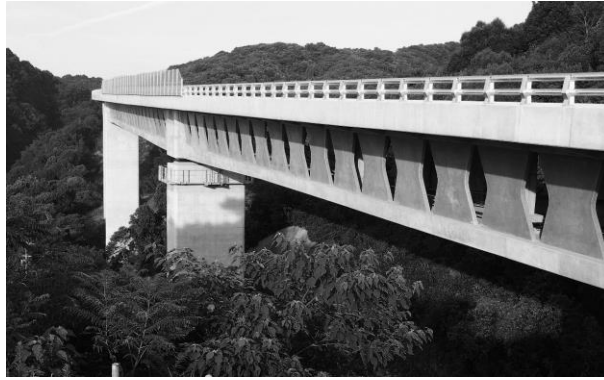
Figure 1. Butterfly web bridge
