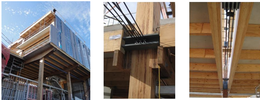
Figure 21. College of Creating Arts - MacDiarmid Building, Massey University, Wellington, New Zealand. Post-tensioned timber (Pres-Lam) frames with draped tendons in the transverse directions with horizontal U-Shape flexural plate dissipaters on the first floor and Post-tensioned concrete (PRESSS) walls in the longitudinal direction (Structural Engineers: Dunning Thornton Consultants)
