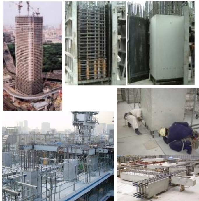
Figure 6. 2000' Precast concrete system (Site PCa)
