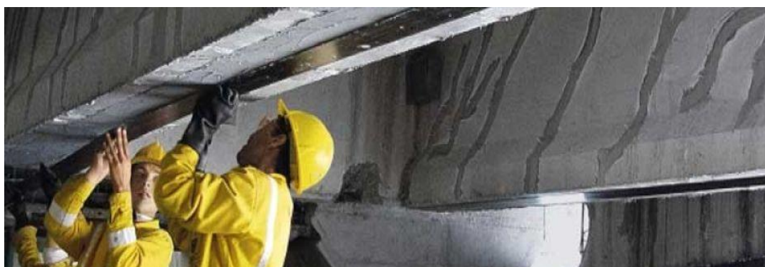
Figure 8. fib MC 2010 model for bending extended for assessment of existing structures or for design of new structures or interventions on existing structures. Use of non-metallic reinforcement.
