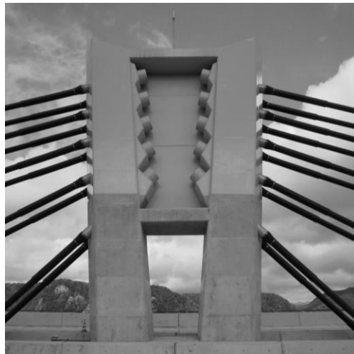
Figure 16. Extradosed cable anchorage of pylon
