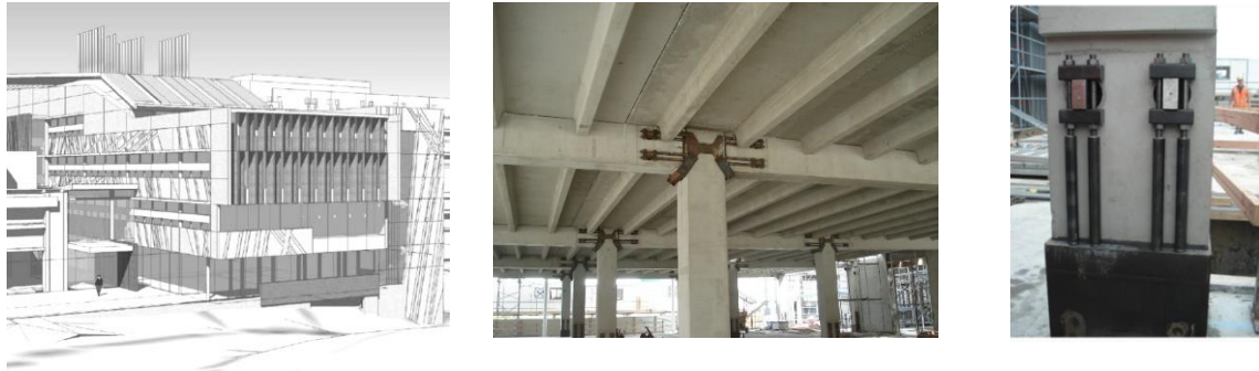
Figure 17. First multi-storey PRESSS-concrete building in New Zealand. Post-tensioned frames with external Plug&Play dissipaters in one direction; Post-tensioned walls coupled with steel beams in the other (Structural Engineers: Dunning Thornton Consultants; Cattanaach and Pampanin, 2008).
