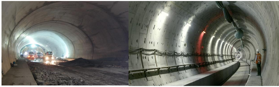
a) Tunnel lining (Riva Railway) b) Precast panels (courtesy of Mehmet Yerlikaya)
