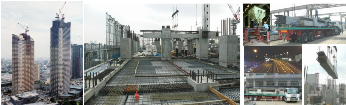
Figure 7. Park city Musashi Kosugi (59F,47F, 2006) using advanced pre-cast concrete system
