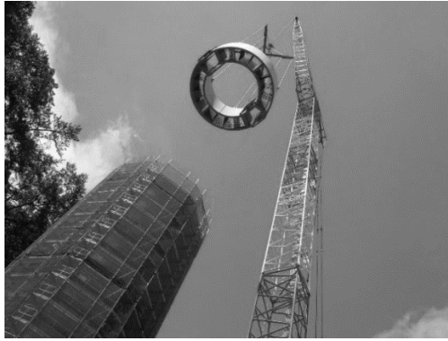
Figure 15. Precast construction of piers
