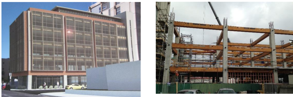
Figure 23. Merritt Building, Victoria Street, Christchurch. Three Storey commercial Building consisting of Post-tensioned timber (Pres-Lam) frames with Plug&Play external dissipaters in the transverse direction and cast-in-situ reinforced concrete wall in the longitudinal direction. (Structural Engineers: Kirk and Roberts; Architects: Sheppard and Rout)
