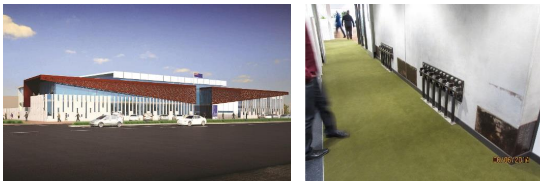
Figure 19. Police Station in Rotorua. Post-tensioned concrete (PRESSS) walls with external & replaceable dissipaters in both directions (Structural Engineers: Spiere)
