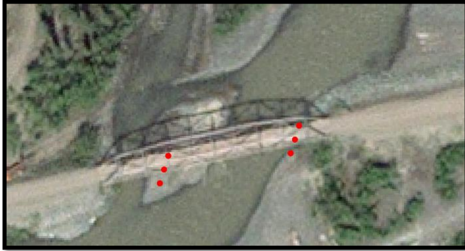
Figure 6: Lakina River Bridge piers represented by red dots.
