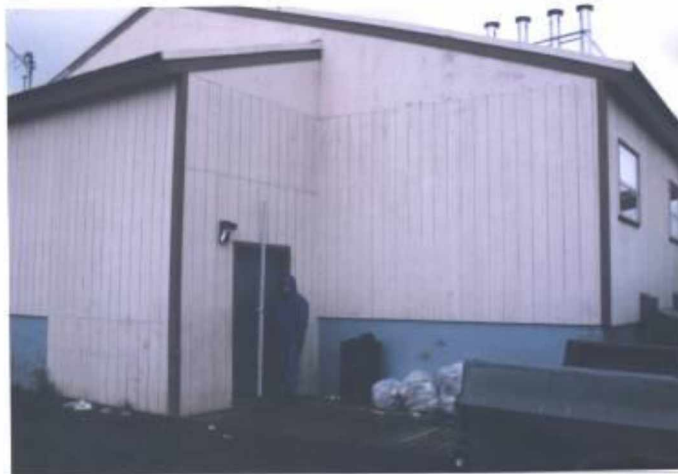
Temporary bench mark is the front door sill at the city hall.
