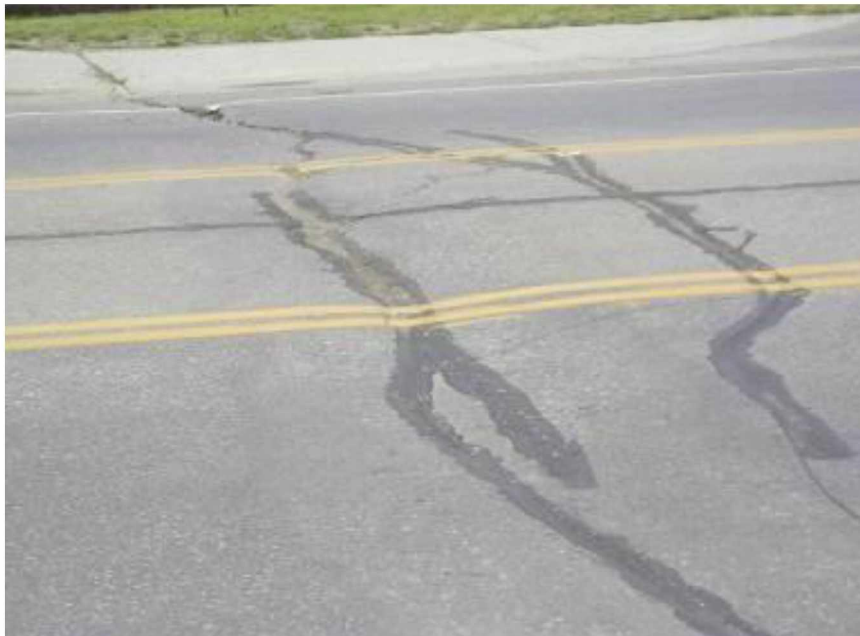
Figure 3.5: South Cushman Street, Fairbanks, crack seal, 2011.
