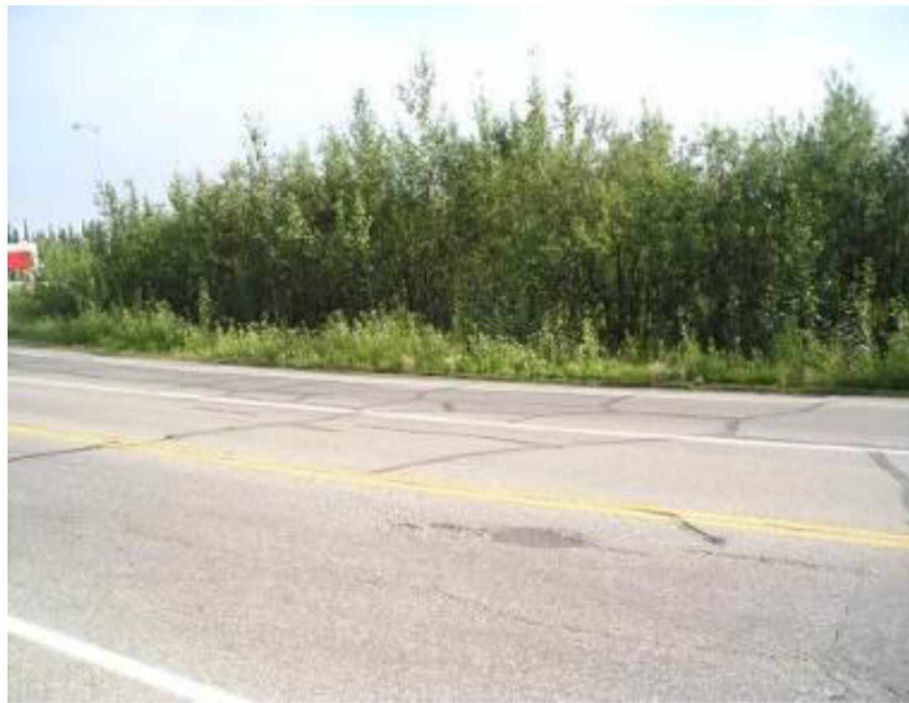
Figure 3.3: Wembley Ave, Fairbanks, crack seal, 2011.
