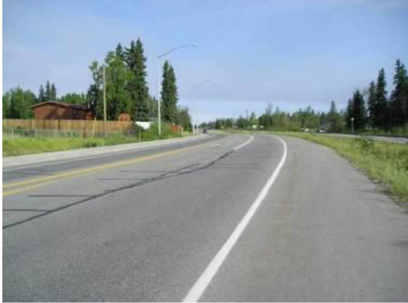
Figure 3.4: Trainor Gate Road, Fairbanks, crack seal, 2011.
