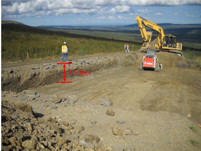
Figure 3.1 Excavation of East Lane (Looking North)
