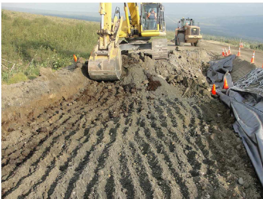
Figure 3.6 Excavation of West Lane of Road
