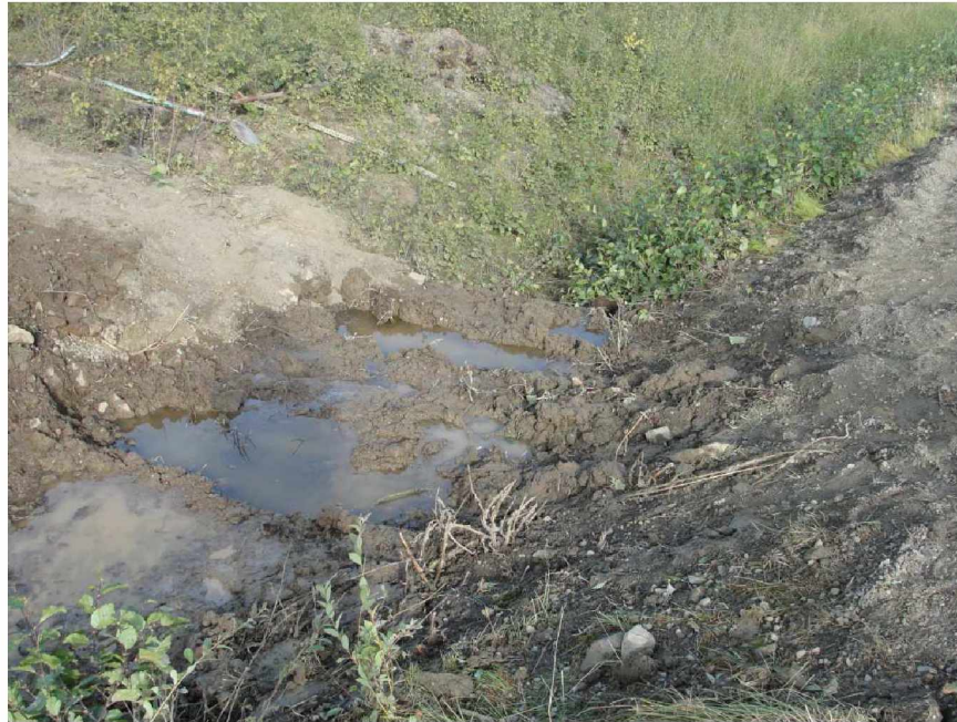
Figure 3.12 Water in Existing Ditch on East Side of Road on August 5, 2010
