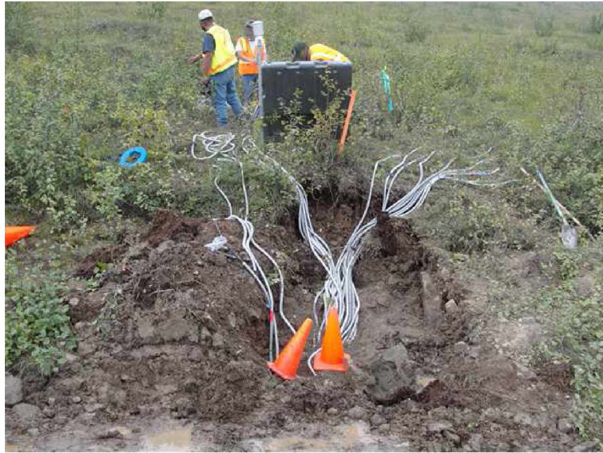
Figure 3.9 Construction of Data Collection Station
