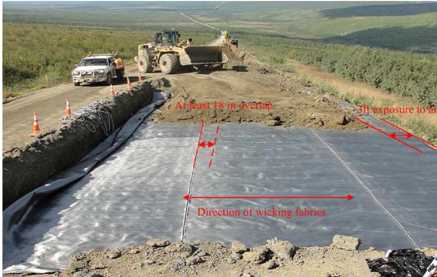
Figure 3.4 Bottom Layer of Wicking Fabric after Placement
