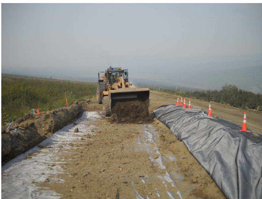
Figure 3.7 First Layer of Wicking Fabric on West Side of Road
