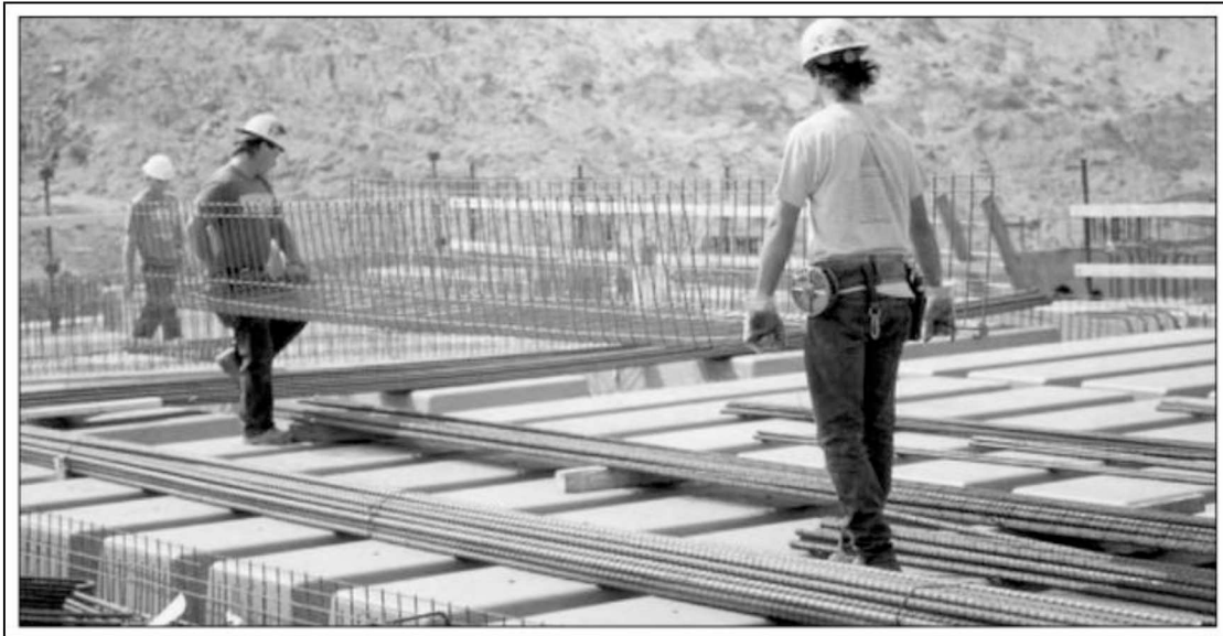
Figure 1.1: Welded Wire Reinforcement for Concrete Girders (Wire Reinforcement Institute 2006)
