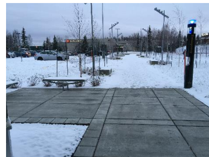
Picture 1: CFT Technology installed at UAA's new engineering building.
