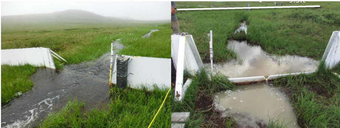
Figure 2.5 Images of the Imnavait Creek weir.
