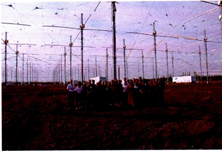
Figure 5.2 HAARP phases array transmitter
