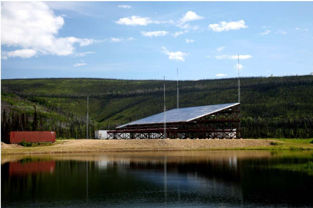
Figure 3.2: Northward looking UHF phased array radar at Poker Flat, near Fairbanks, Alaska.
