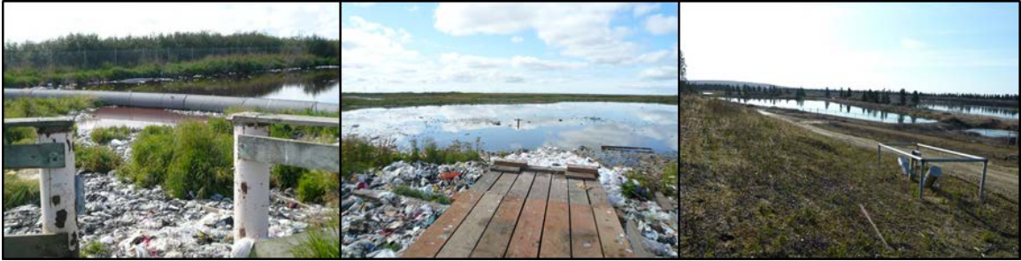
Figure I-4: Illustration of rural Alaska unmanaged (right) and managed (left) constructed and non-constructed natural honeybucket (mid) sewage lagoons.
