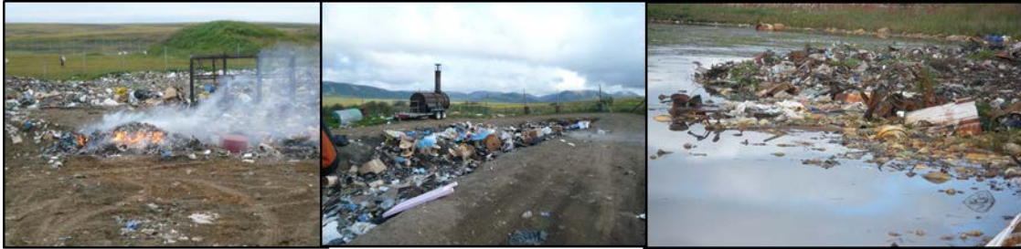
Figure I-1: Illustrates the three most common landfill designs in rural Alaska (left) above ground; (mid) trench-filling; and (right) tundra pond.
