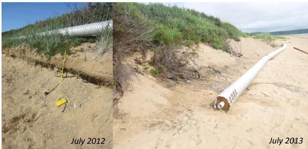
Figure 2.8—Pipe located on actively retreating bluff toe on south side of the Golovin sand spit, at Profile 1.
