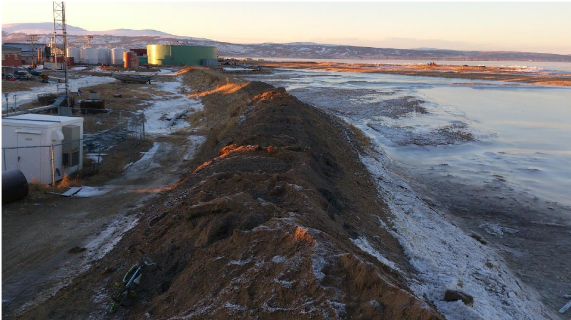
Figure 4.16—Temporary levee constructed before November 2013 storm, photo by Carol Oliver.
