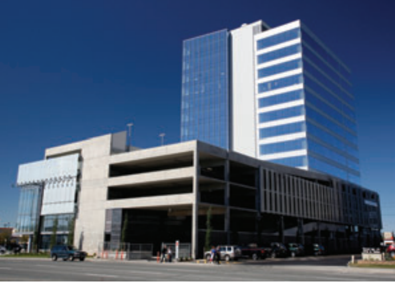
188 West Northern Lights, Anchorage
