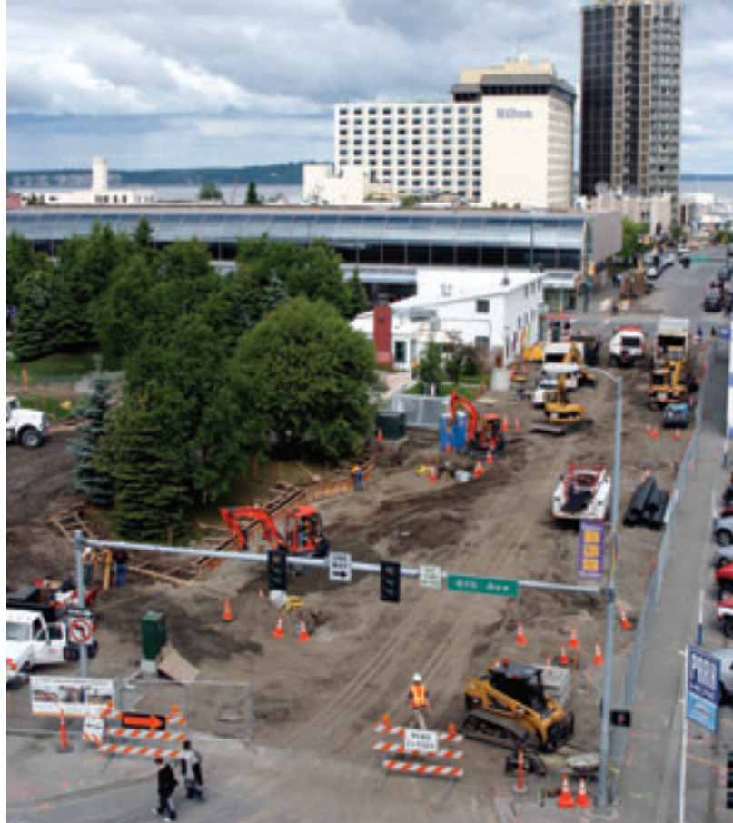
E Street Improvements, Anchorage
