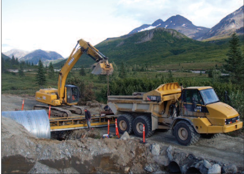
PHOTO COURTESY NORTH STAR PAVING
