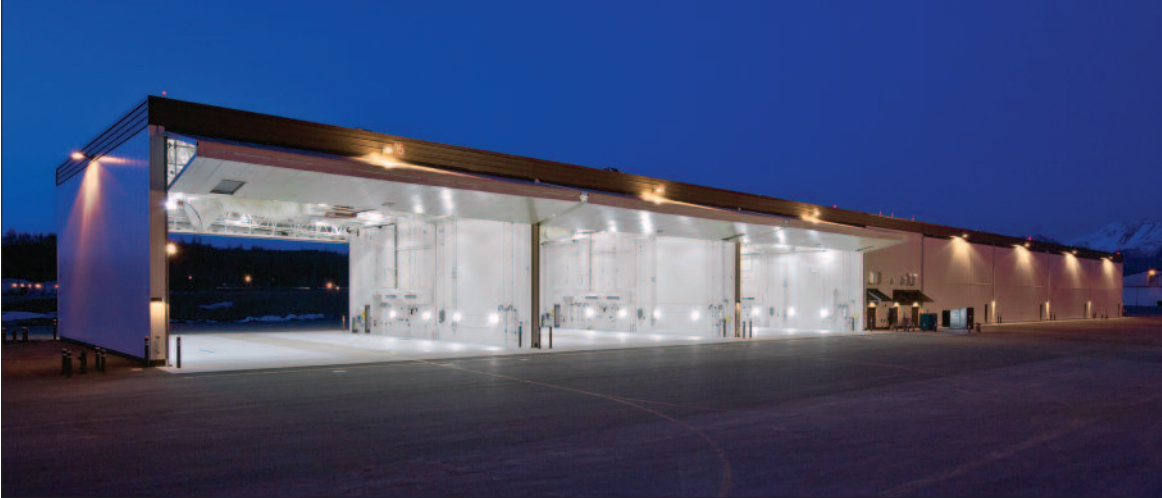
PHOTO BY KEN GRAHAM COURTESY KIEWIT
