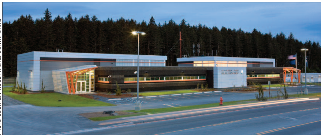
PHOTO COURTESY ROGER HICKEL CONTRACTING
