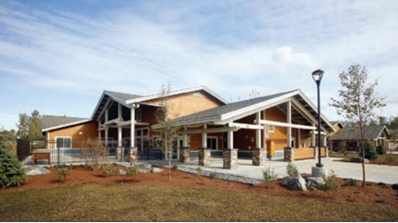
Providence Extended Care Facility, Anchorage, Davis Constructors and Engineers, Inc.
