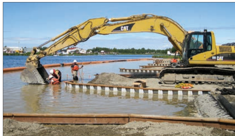
Lake Hood Bank Stabilization, Anchorage, Granite Construction
