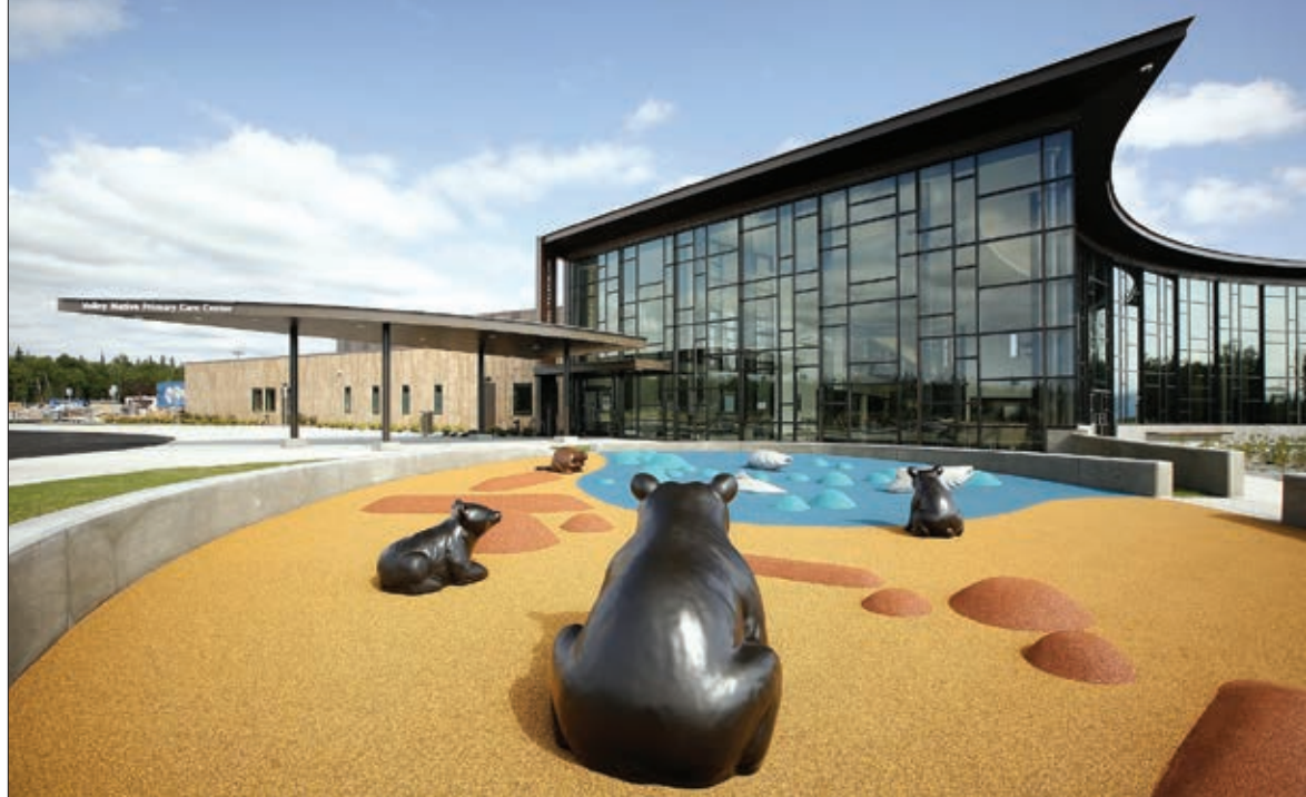
Valley Primary Care, Wasilla, Neeser Construction
