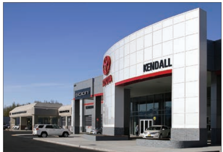
Kendall Auto Dealership, Anchorage, Brady Construction
