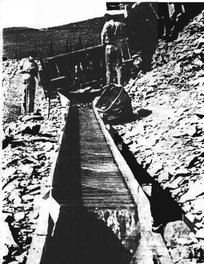
Figure 14. Sluice Box at Mine No. 2
