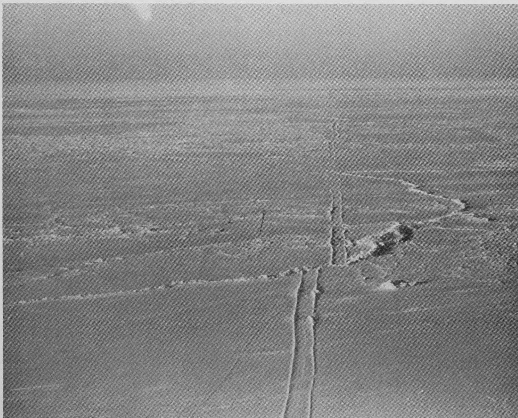
Figure 6. Seismic line ice road displacement (center section) west of Narwhal Island in March 1979.
