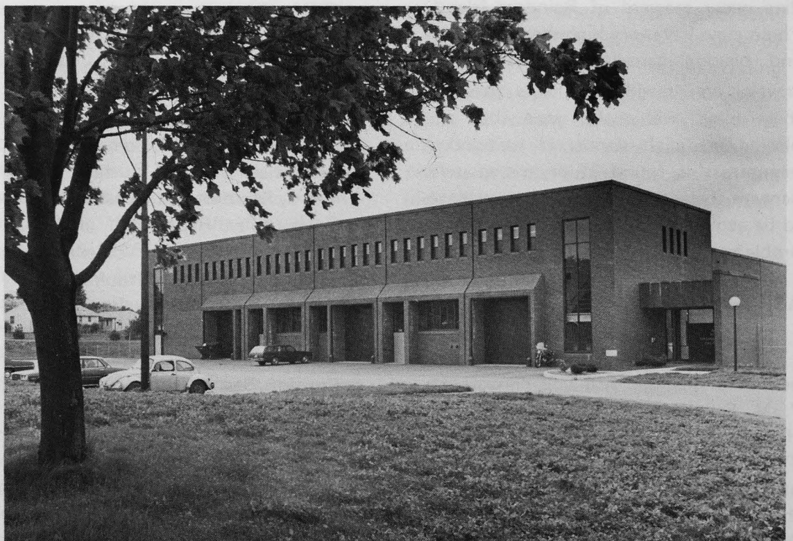
CRREL's Ice Engineering Facility.
