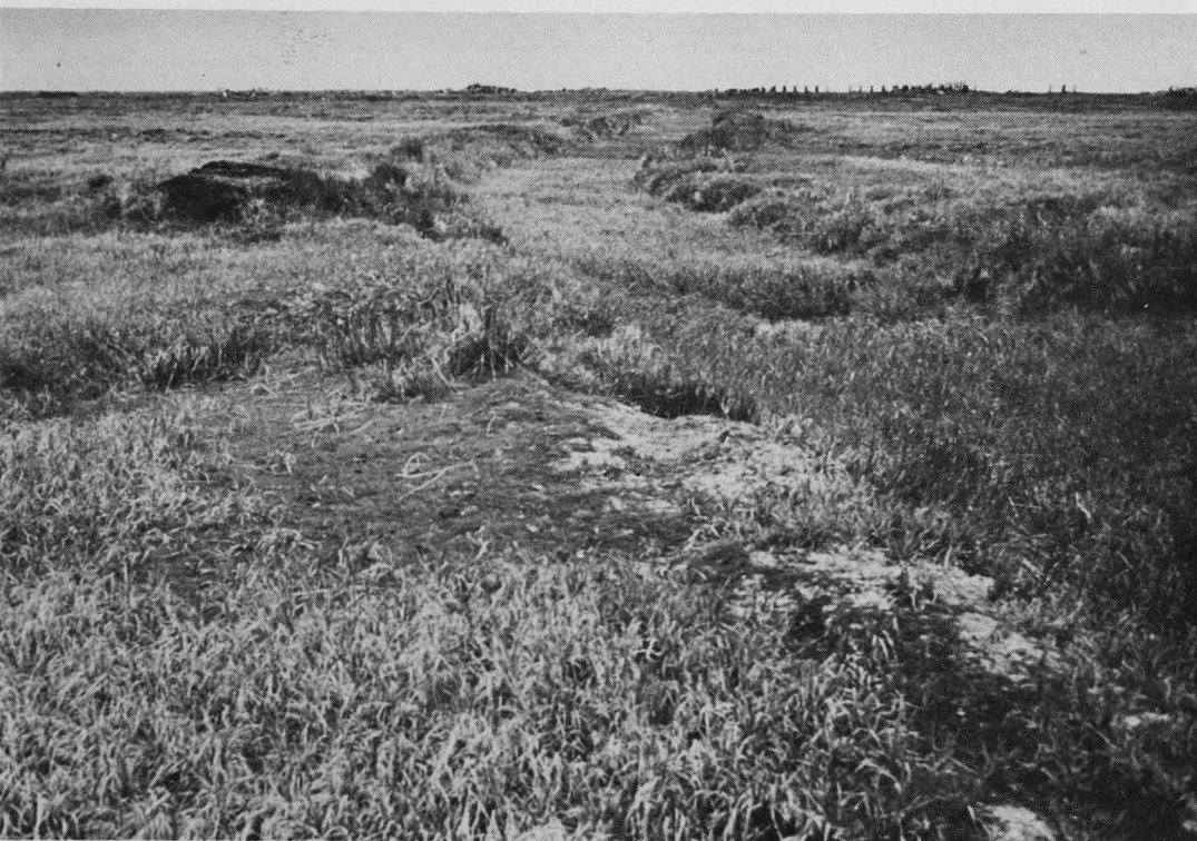
Figure 4. A bulldozed trail with berm at the Fish Creek drill site. A small thermokarst pond lies in the trail, near the center of the photo. View is northeast toward the drill site.
