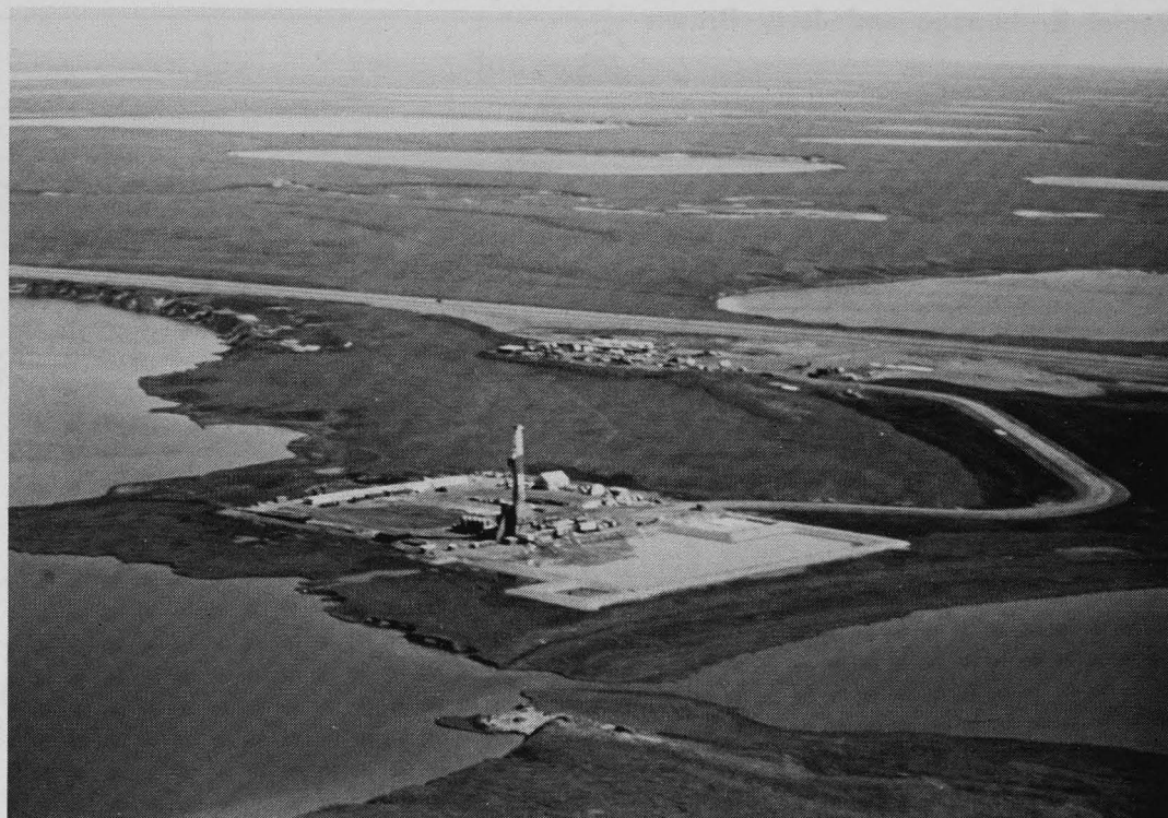
Figure 4. Aerial view of completed airfield and drill site at Inigok, July 1978.
