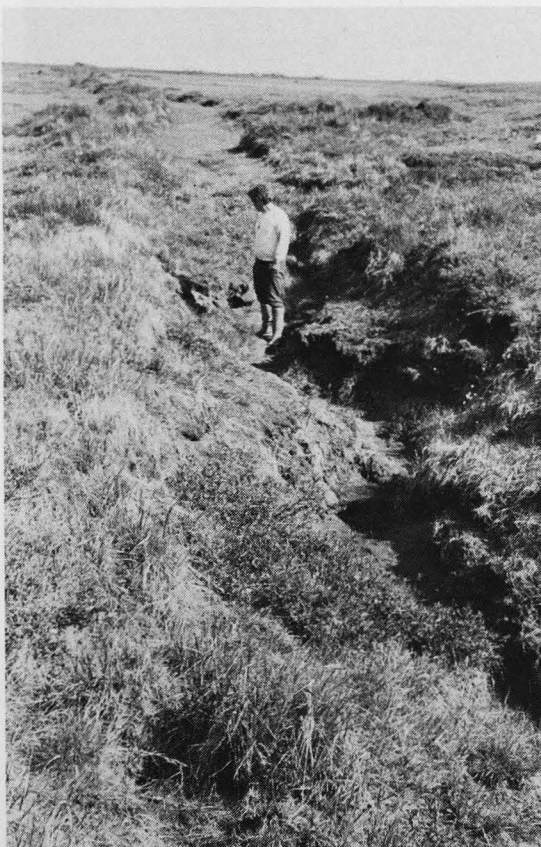
Figure 7. Gully formed by thermal and hydraulic erosion along a thermokarsted, bulldozed trail at the Fish Creek drill site.
