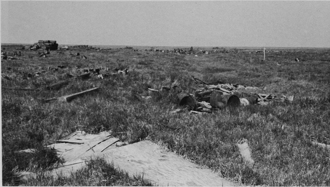
Figure 5. Wood, 55-gallon steel drums and other debris littering Fish Creek site. A large stack of steel drums lies near the horizon, left of center. Below it, short wooden piles protrude above the vegetation.
