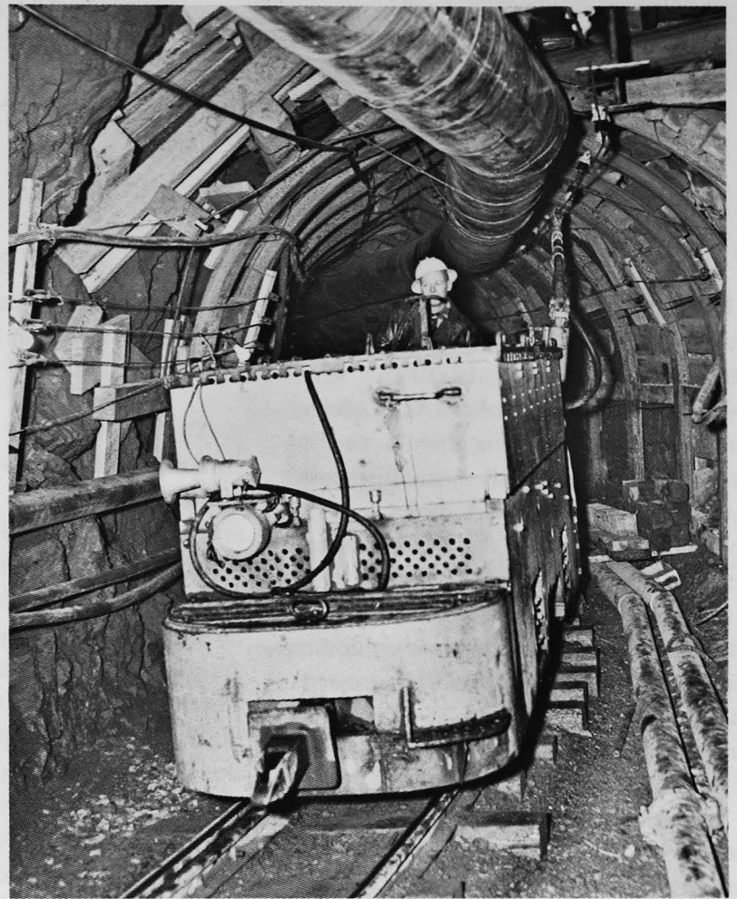
A battery-driven locomotive inside the Eklutna tunnel, a 4 1/2-mile long bore driven through the Chugach Mountains.
