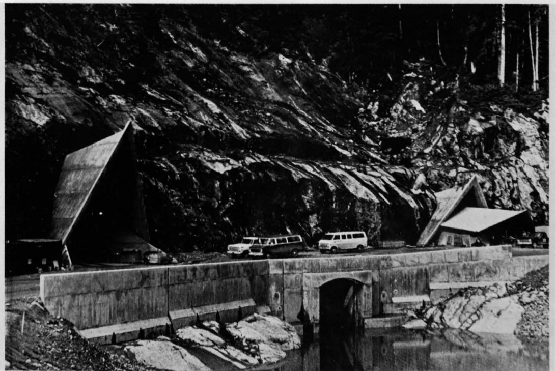
Figure 10. Powerhouse entrances, left to right: access tunnel, tailrace tunnel (below vehicles), service tunnel.
