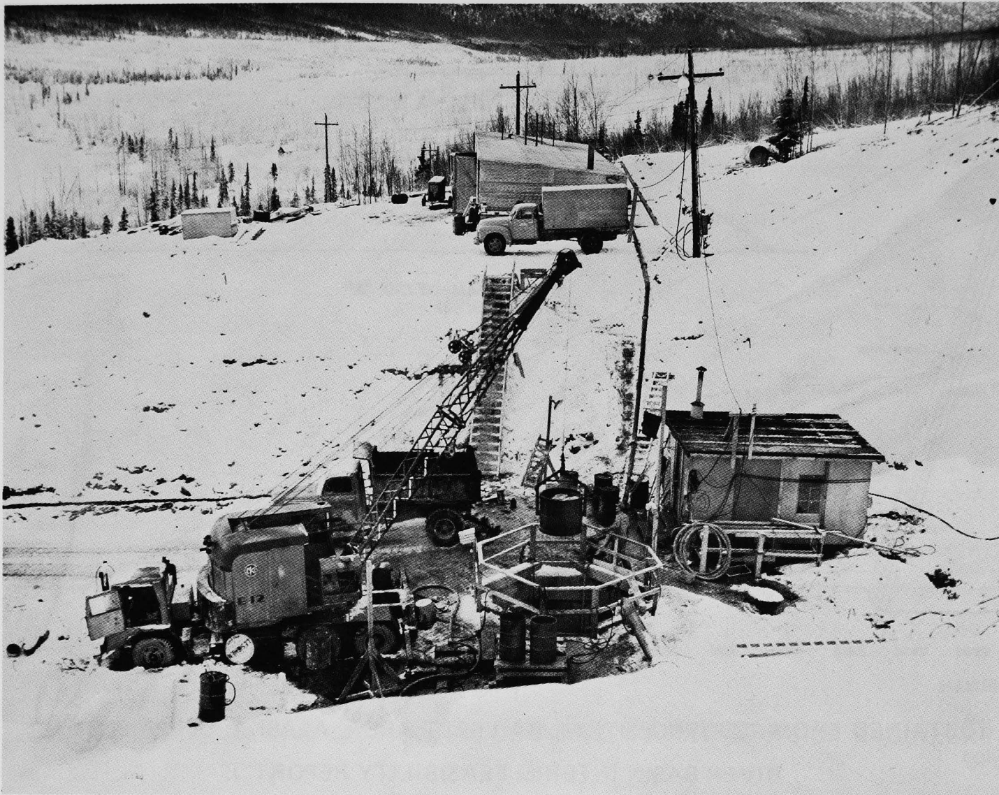
Work underway on the gate shaft.
