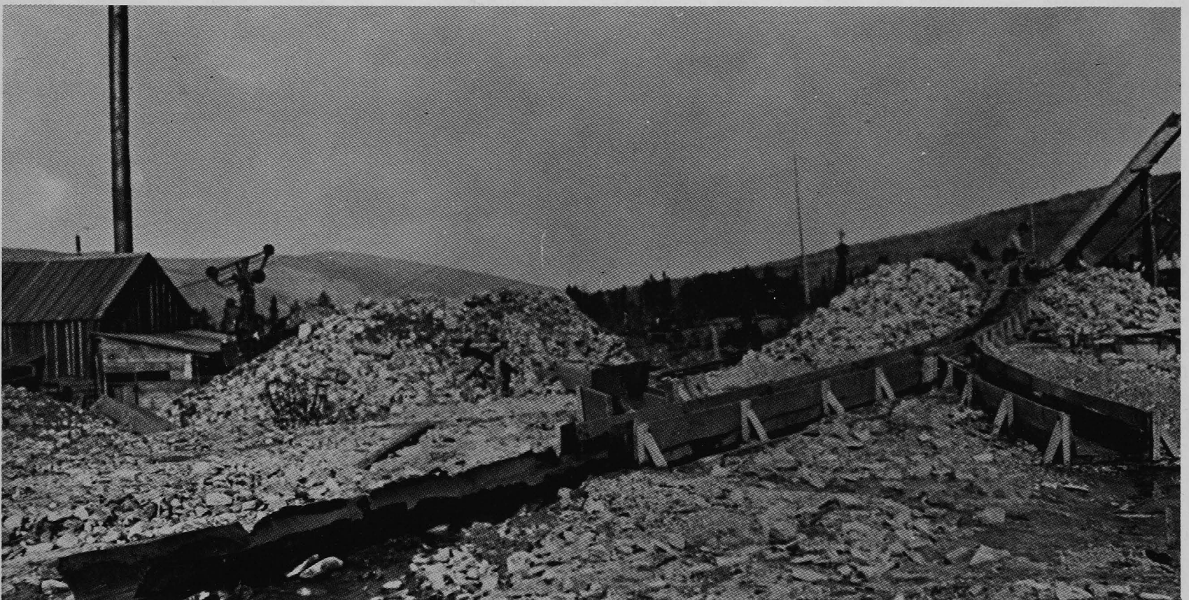
An unusual Y-shaped sluice; "arms" were built onto the sluice to divert tailings as needed. (Courtesy of Selid-Bassoc Collection, Archives, University of Alaska, Fairbanks.)
