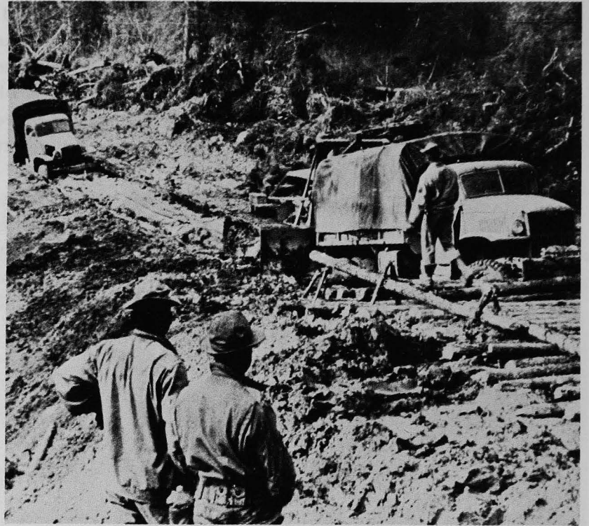
Pushing and/or pulling foundered trucks along the muddy pioneer road was a continuing assignment for roving tractors.
