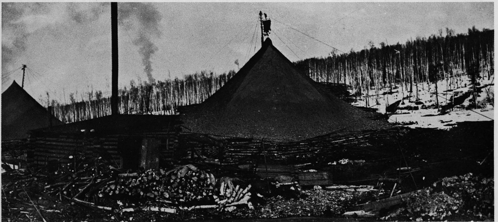
A huge bucket dumps its load onto a mound of gravel awaiting sluicing. The log structure covers an underground shaft. Wood-powered boilers provided steam for thawing. (Courtesy of Charles Bunnell Collection, Archives, University of Alaska, Fairbanks.)
