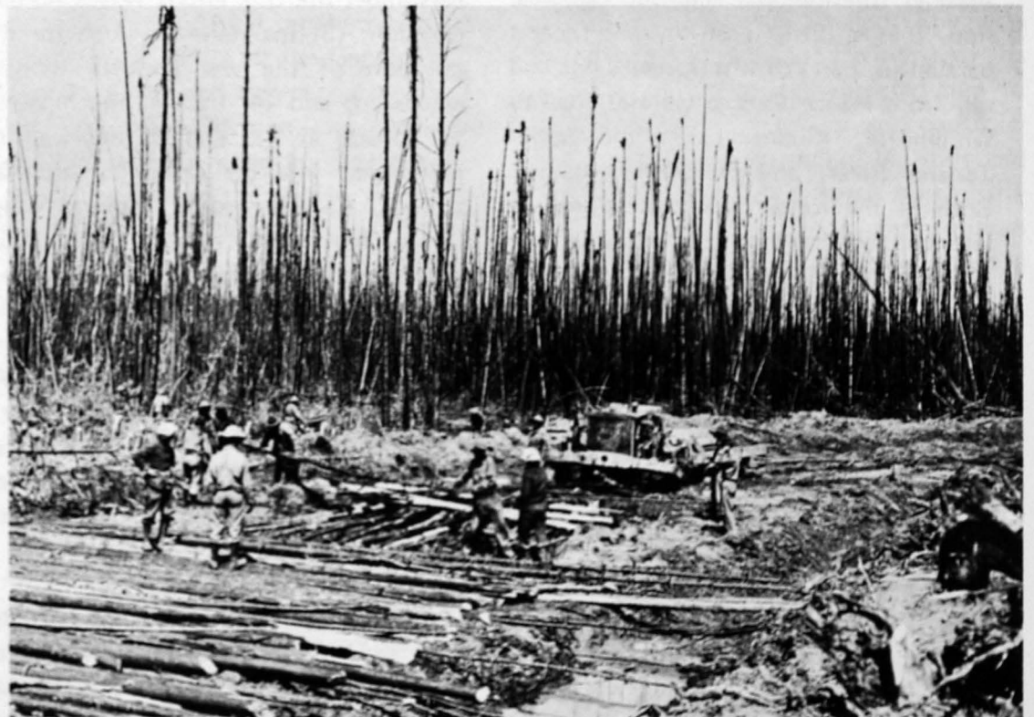
In muskeg areas, layers of timber gave a corduroy road base that was covered with dirt. Plenty of straight timber was found in forests burned years earlier.
