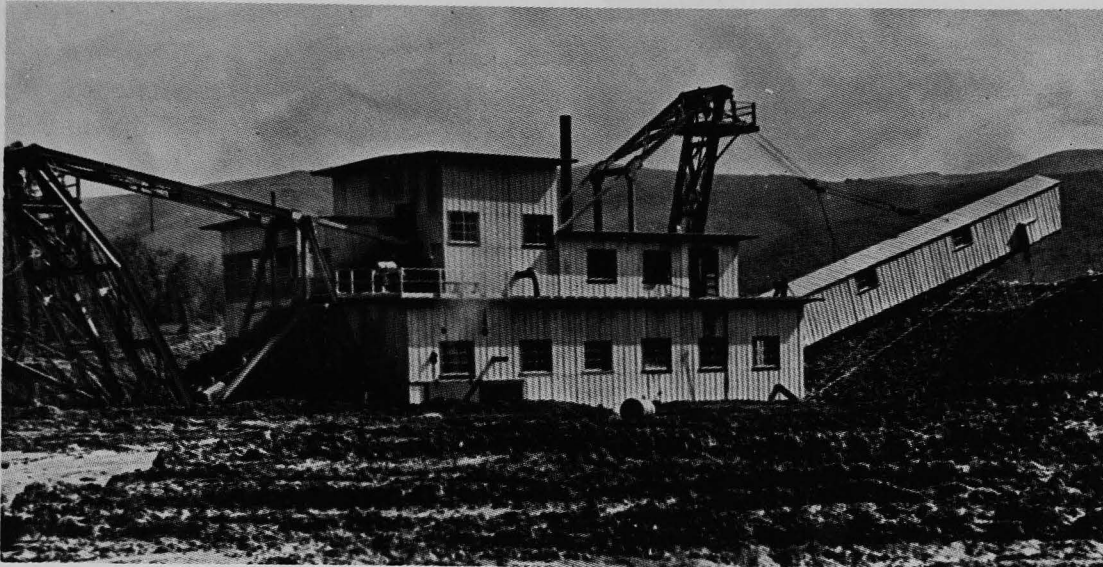
An example of the type of gold dredge operated in the Forty-Mile district. This method was much more profitable than panning and sluicing. Note the ridges of tailings in the foreground. (Courtesy of Mike Erceg Collection, Archives, University of Alaska, Fairbanks.)
