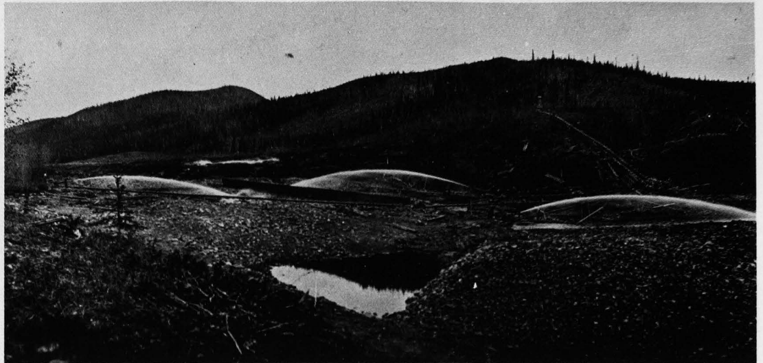
An example of hydraulic mining as used in the Forty-Mile; great jets of water were used to strip away the overburden. (Courtesy of J. S. Norwood Collection, Archives, University of Alaska, Fairbanks.)
