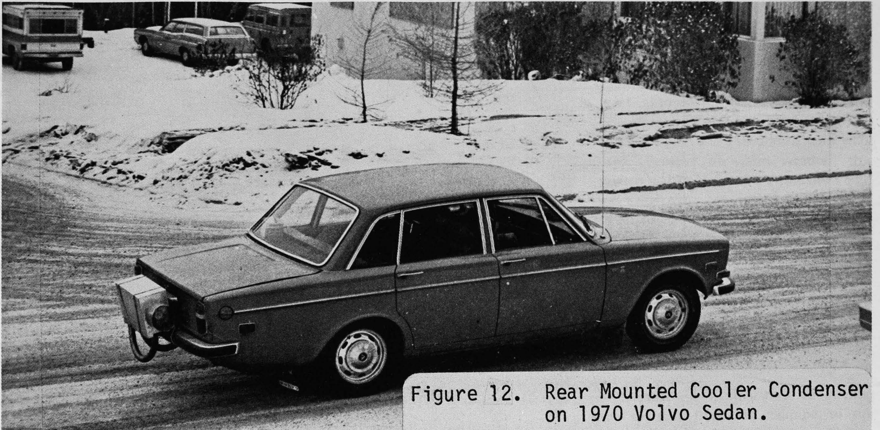
Fig. 12 Rear-mounted cooler-condenser on 1970 Volvo sedan.
