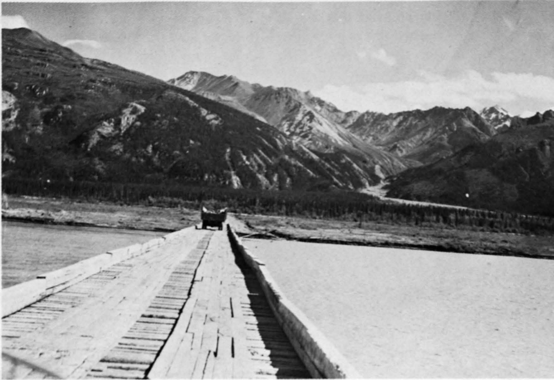
Original bridge at Kluane Lake.
