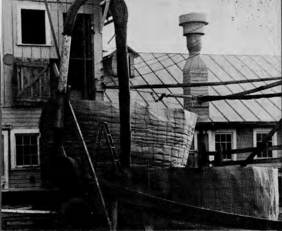
Figure 7. Temporary silos are made from fence and sisal-kraft paper.
