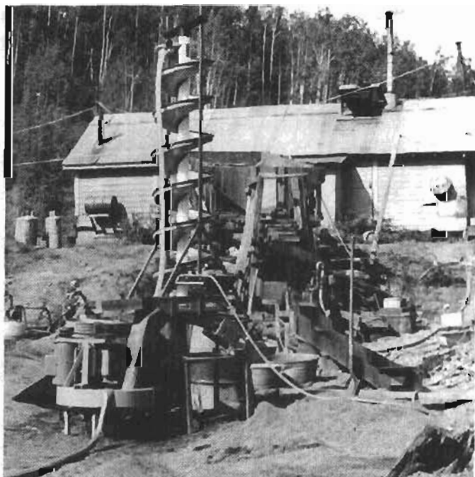
Figure 6. Portable spiral pilot plant being tested at Coal Creek, Alaska.
