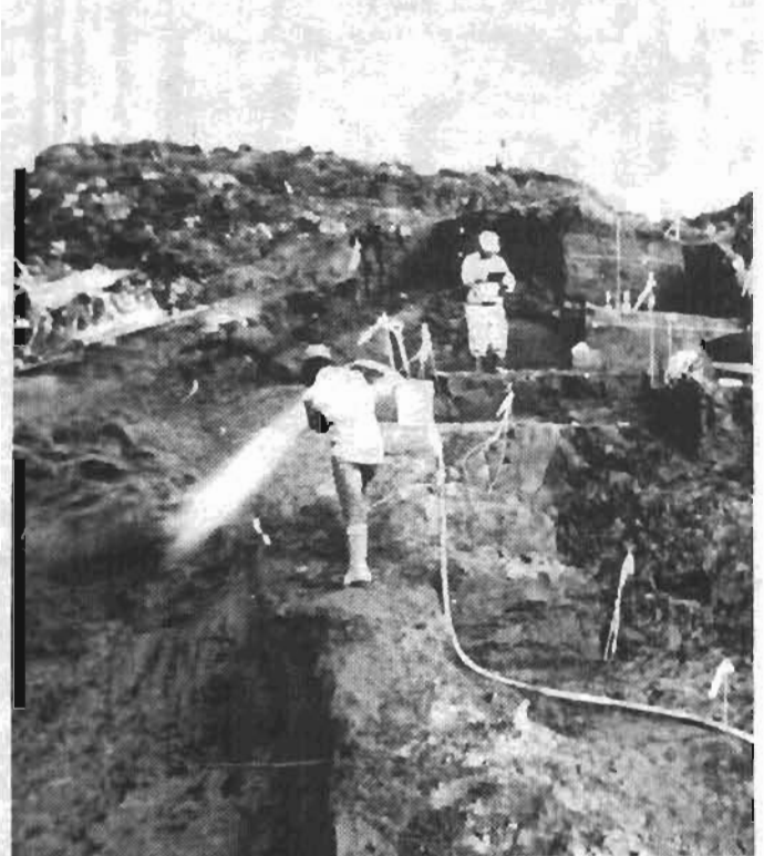
Figure 11. Using hydraulics to excavate the area.
