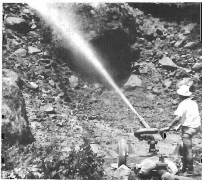
Figure 6. Hydraulicing.
