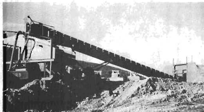
Figure 6. Feeder - conveyor system used in the 1983 mining season.
