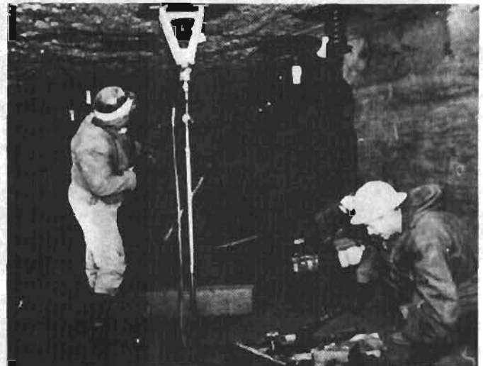
Figure 8. Roof bolt installation.
