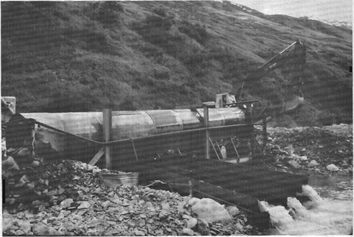
Fig. 4: Trommel washing plant processing placer gravels on Mills Creek, Kenai Peninsula, Alaska, in August of 1980.
