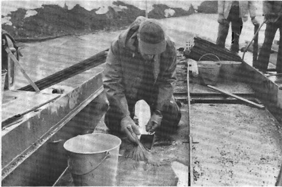
Fig. 16: Final pick-up in the sluice box.
