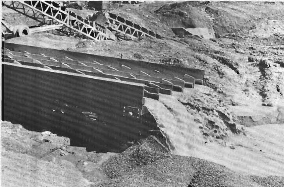
Fig. 10: Discharge of the -\frac{1}{4} " material from the sluice box.
