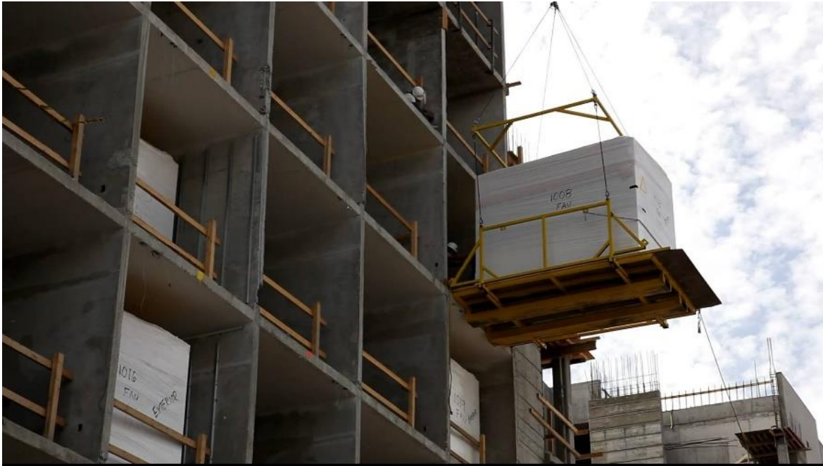
Figure 22 - Prefab bathroom unit installation (Folj 2017).
