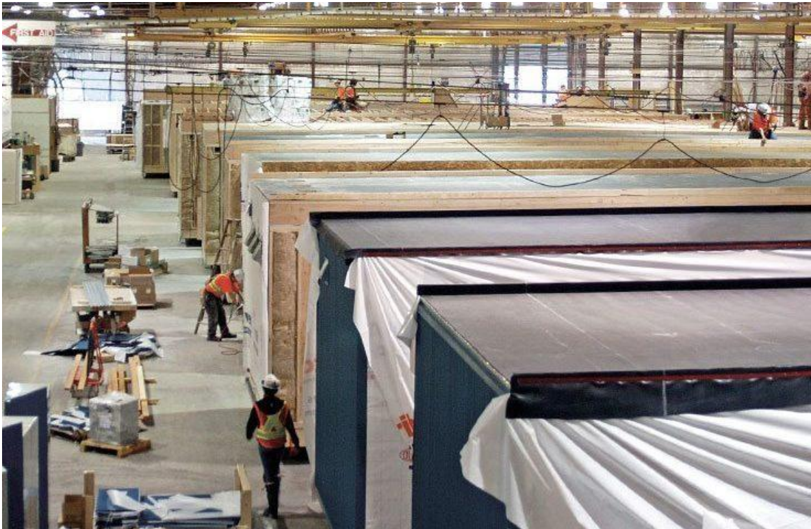
Figure 14 - Off-site fabrication of components manufactured under a controlled environment (Engenharia 2017).
