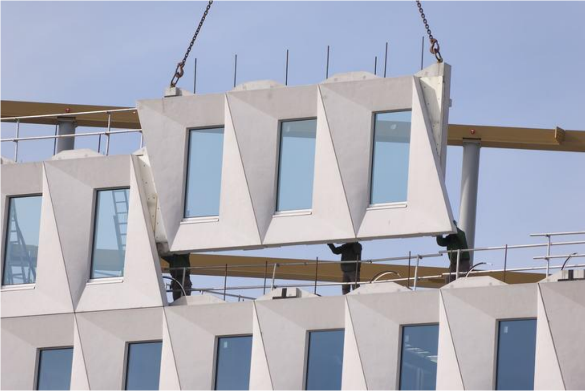
Figure 23 - Prefabricated building blocks' implementation on a construction site (Voordijk and Adriaanse).
