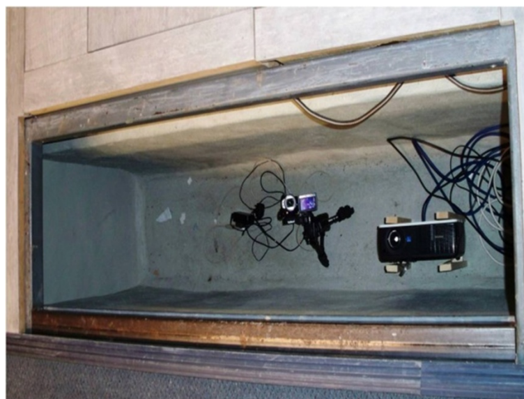
Figure 3 4DFRS. The system consists of a video camera and LCD projector, both embedded in a pit of a dedicated walkway. Picture imaged from above.
