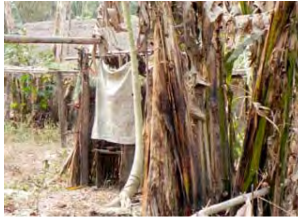
“Toilets” in Nangalbhanga camp in Chirang District, Assam, do not correspond to Sphere standards. (Photo: Anjuman Ara Begum, March 2011)
