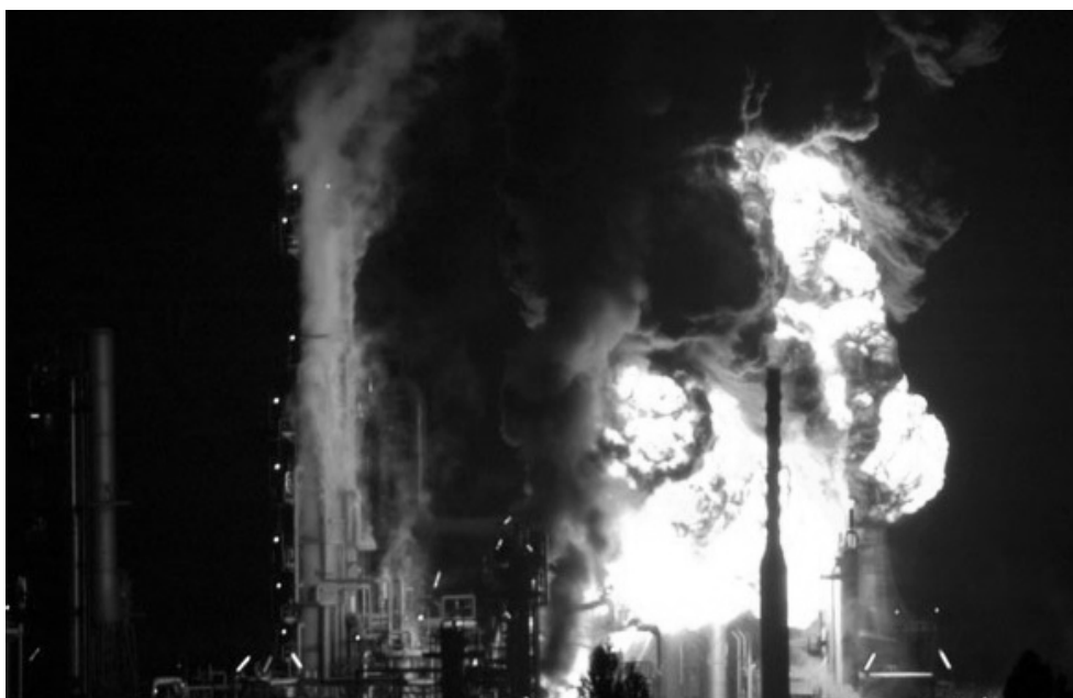
Figure 2: Hydrogen jet fire originated at the Hydrodesulphurization reactor and following accident escalation with fire development of diesel oil in the nearby area.
