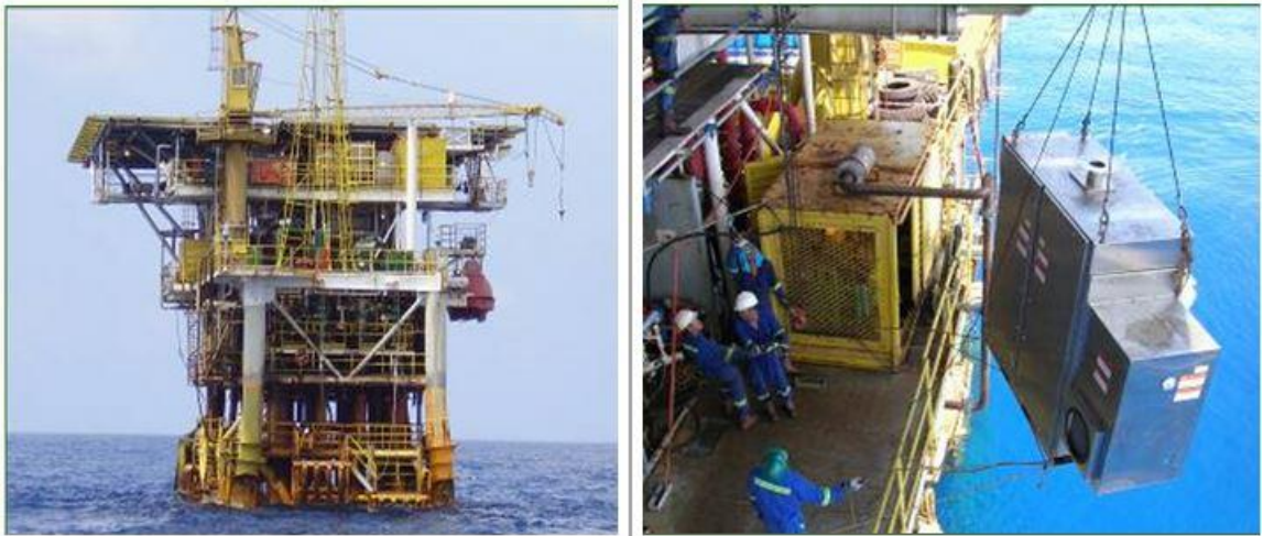
Figure 1: gas turbine plant on platform, Wintershall Holding GmbH
