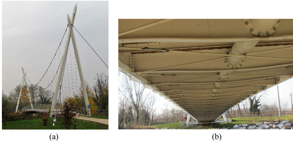
Fig. 5. Seriate Footbridge: (a) overall view; (b) view of the deck; a stabilizing cable is visible on the left.
