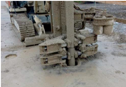
Fig. 9. Execution of micro-pile through the existing piers
