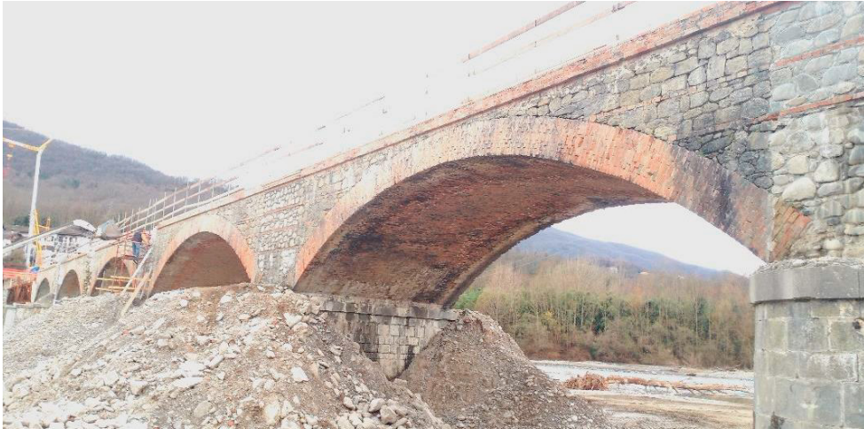
Fig. 18. Restoration of the external surface
