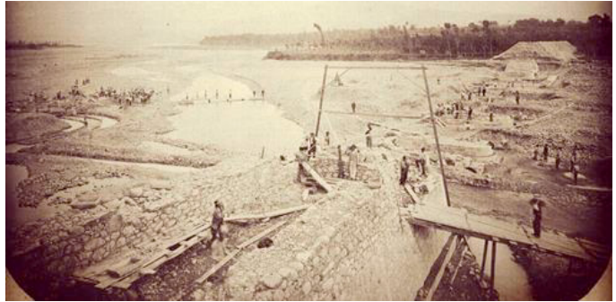
Fig. 2. The Villafranca bridge during the erection phase (1874)
