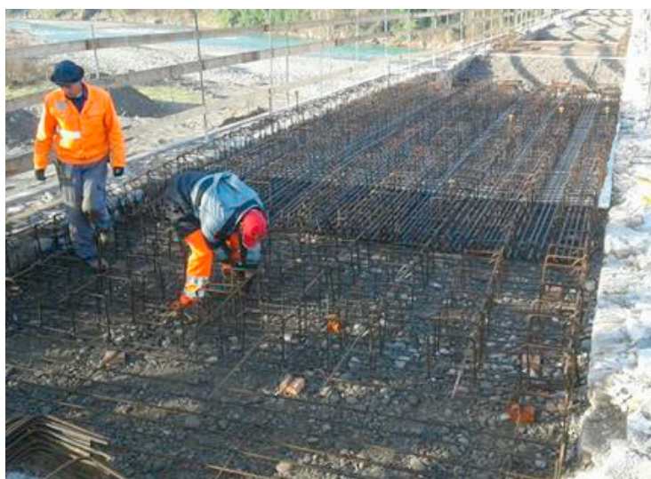
Fig. 14. Preparation of the new r.c. cast in situ deck
