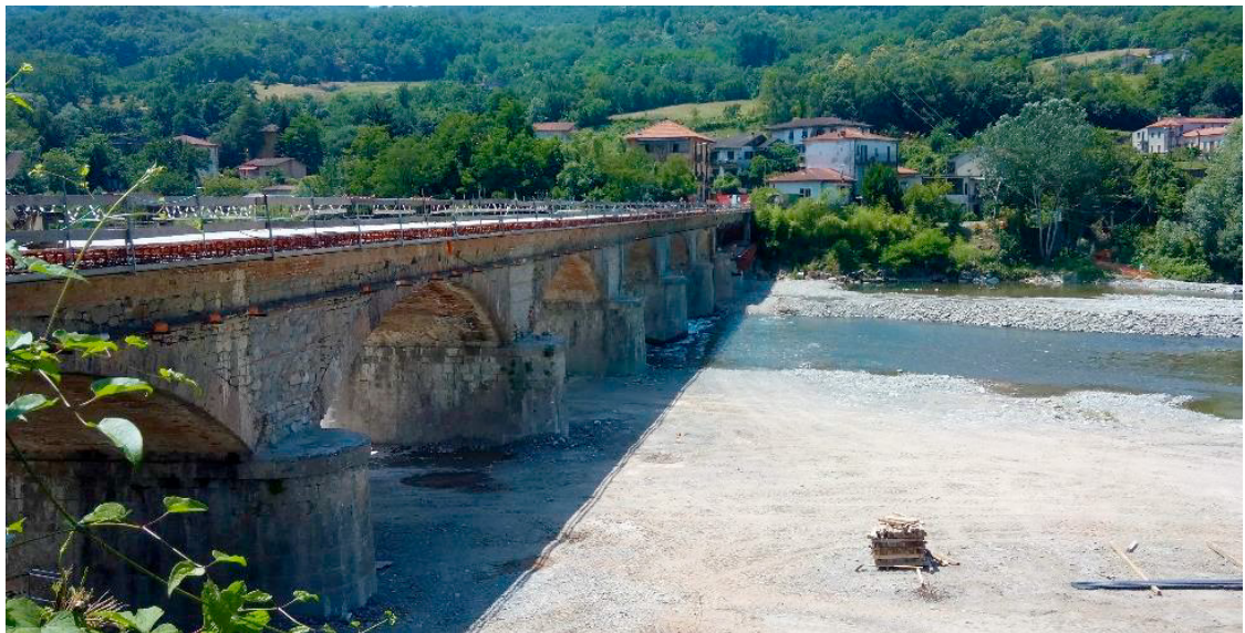
Fig. 17. The bridge after the dismantling of the prefabricated r.c. beams
