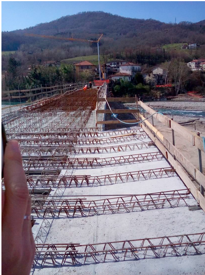
Fig. 19. Preparatory works for execution of the continuous r.c. slab
