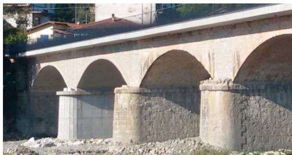
Fig. 7.(a) The new r.c. arches and pier
