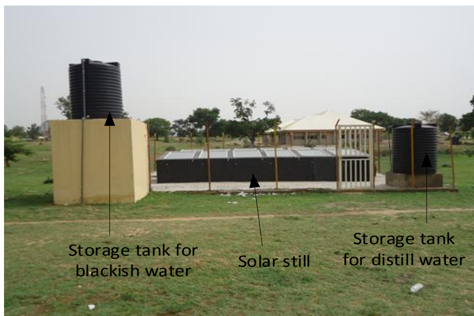
Figure 6 – Pictorial view of the constructed solar still
