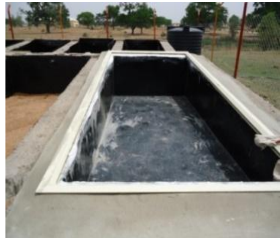
Figure 2 – Still basin: Design and pictorial views of the still basin
