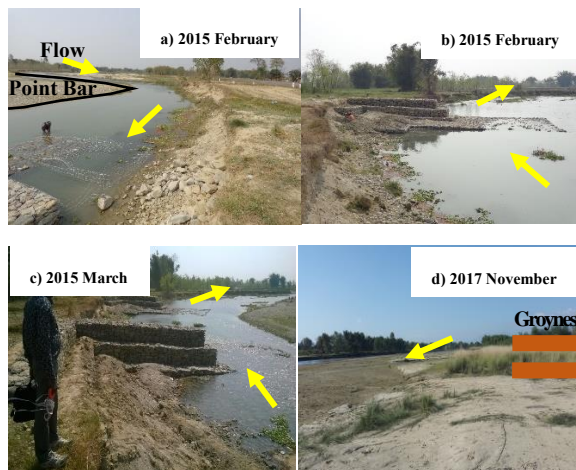
Photo 5: Implementation of groynes in Lohandra River.
